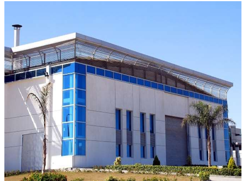
Smart Village, Egypt's first DC project
