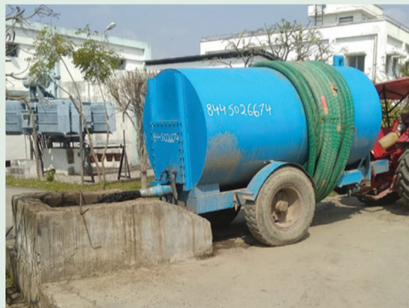
Current practice of direct discharge of FSS at inlet pumping station at Kargi Chowk STP
