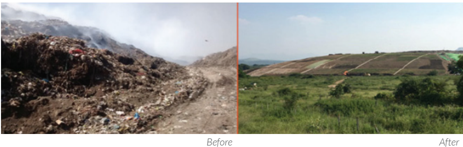
Fig 3.3: Partial land reclamation and capping project in Nashik 1
