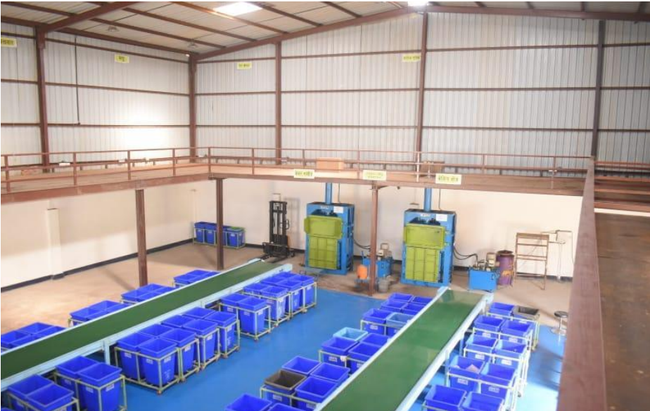
Figure 12: MRF Setup with segregation bay at Zakhira, New Delhi
