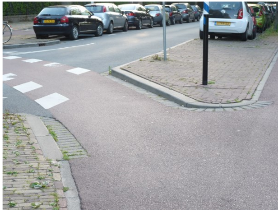
Fig. 3.6 A smooth road surface, also at intersections, leads to better comfort.
