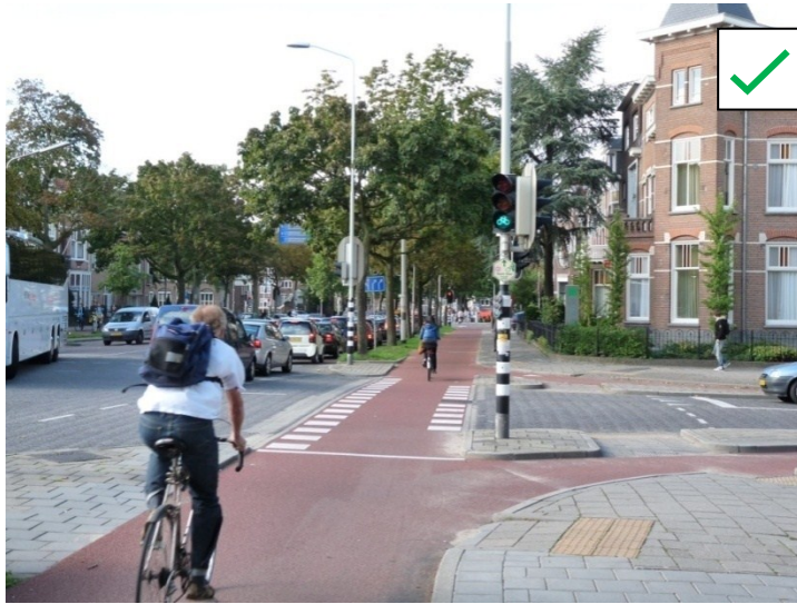
Fig. 3.2 Coherence at intersection level: cycle track is clearly marked across the intersection
