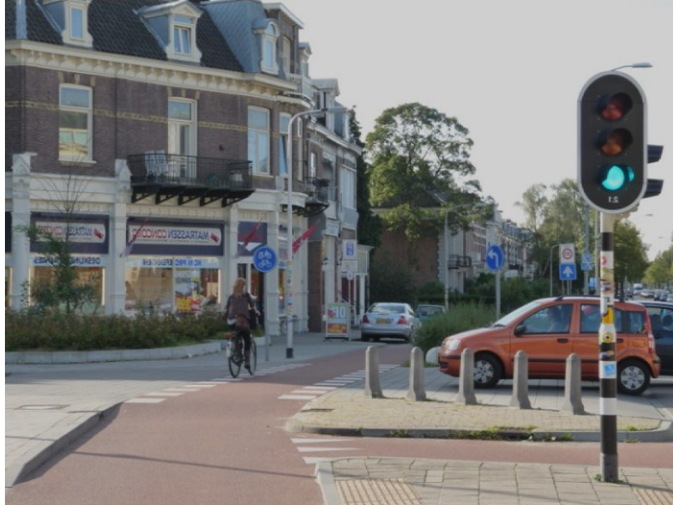
Fig. 6.5 Bending out of an elevated cycle track at side road
