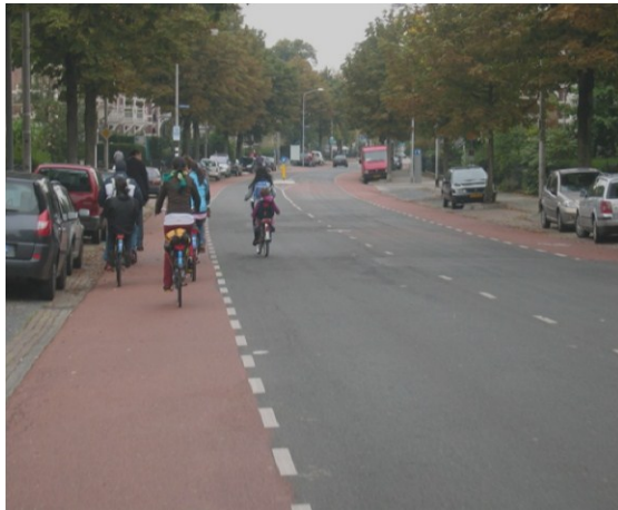
Fig. 4.12 Cycle lanes (1.80 m.) on a collector road in The Netherlands
