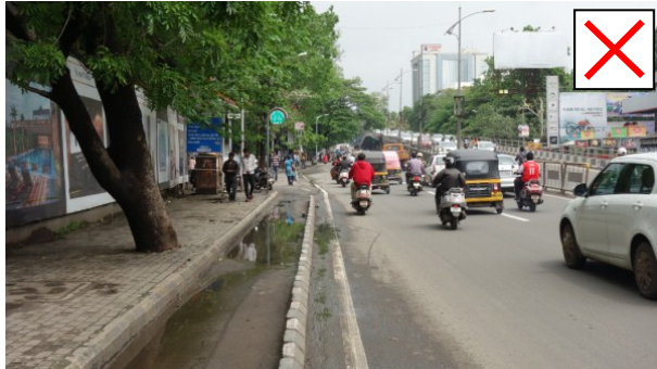
Fig. 4.5a Road level cycle track without proper drainage
