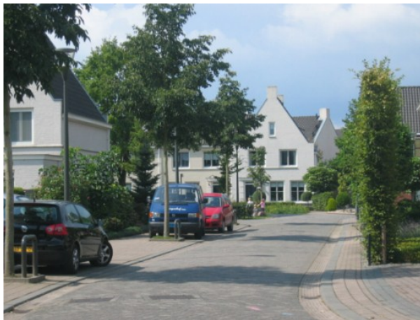
Fig. 4.14a Access Street with shared use and parallel parking bays
