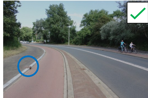
Fig. 4.5b. Road level cycle track with proper drainage
