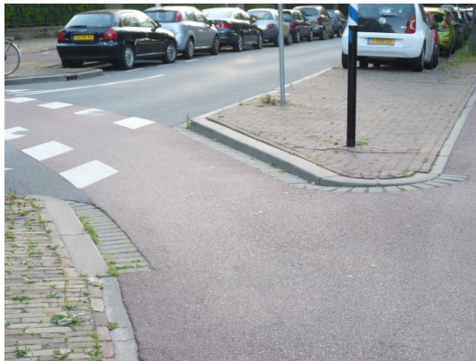
Fig. 7.1 A smooth transition between a raised cycle track and the carriageway
