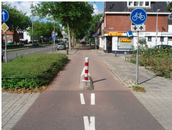
Fig. 7.9 A narrow two-way cycle track with a bollard
