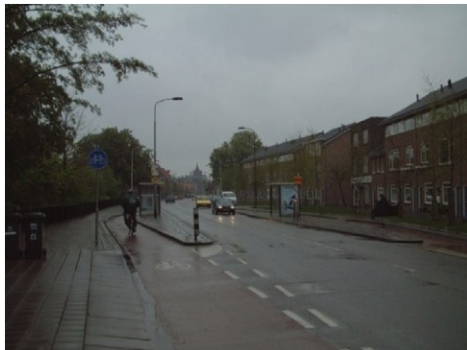
Fig. 7.7 Cycle lane converts into cycle track behind bus stop / bus shelter.
