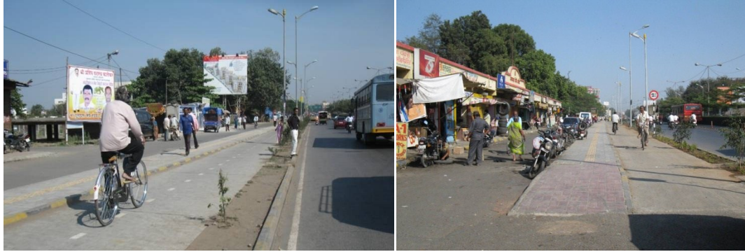
Fig. 4.8 Two-way cycle track with raised footpath and green verge at Solapur Road (Pune)
