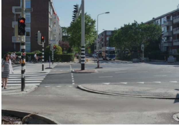
Fig. 6.8 Segregated design at intersection with one-way cycle tracks
