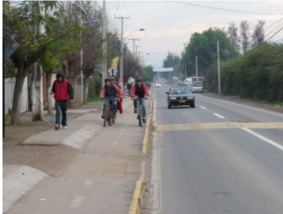
Fig. 3.4 Lack of road safety at road section level. This cycle track is too narrow.
