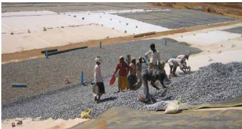
Figure 4.13: Sanitary Landfill under Construction 17
