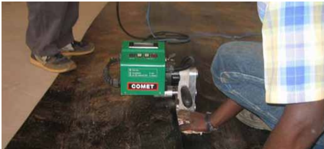
Figure 4.17: Proof of welding seams 21
