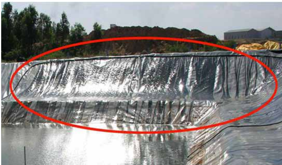
Figure 4.11: Irrigation of Leachate on the Slopes of the Pond. 15
