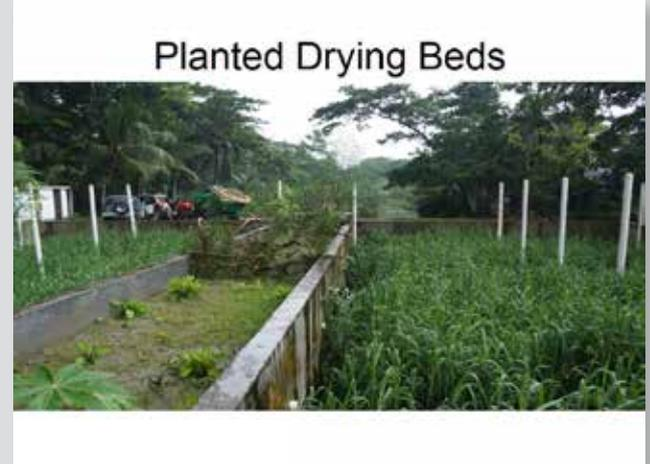
A planted drying bed is a type of drying bed which uses plants (macrophytes) to stabilize and dewater the sludge.
