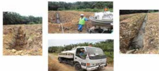
Trenching is a simple technique in which the faecal sludge is buried as a temporary option.
