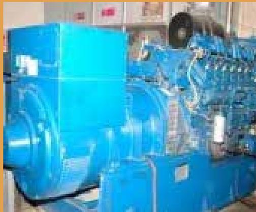
Biogas engine for power generation, Nessapakkam STP
