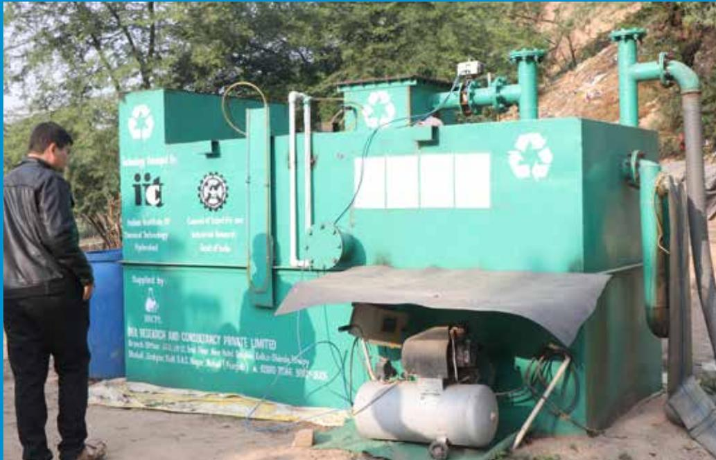
temple has installed a composting Organic Waste Converter (OWC) of 30 kg capacity in 2016. The compost produced here is being used for horticulture purposes. Only one person is required to operate this facility.
