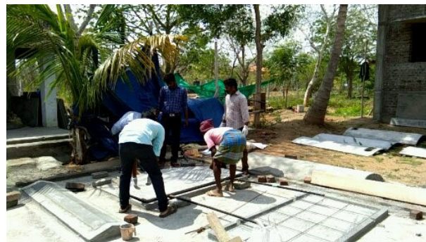
6 Joining slab mould and doors at platform
