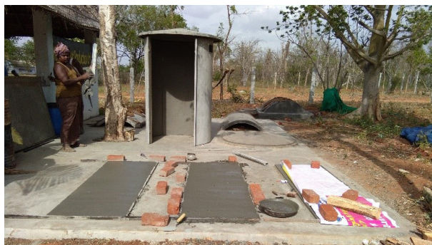
5. Slab curing for doors
