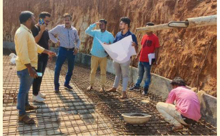
Interns working at site Rayagada, Odisha
