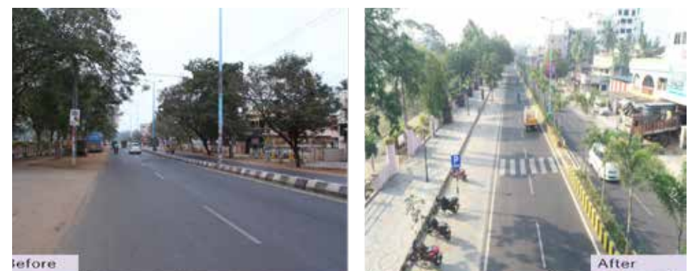
Figure - 11 Before and After Execution Pictures at Boat Club
