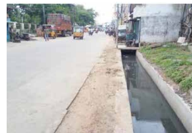
Figure - 4 Uneven Pedestrian Surface with Obstructions
