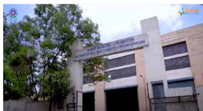
Figure 1: SMAC Centre, Source: Surat Smart City
