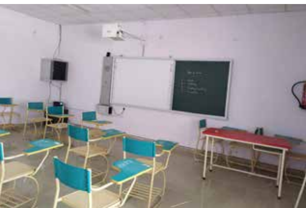
Figure-5: E-pathshala installation status in Shri Kailash Nath Balika Inter College, Civil Lines. Source: Author
