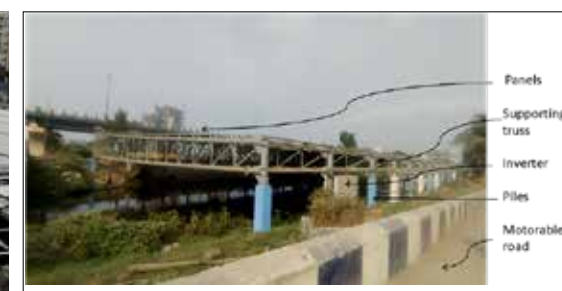
Fig. 4. View from the canal side road of the installed 500kW solar PV plant parts Source: Author
