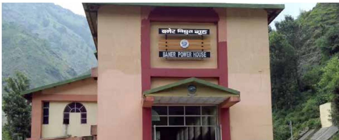
Figure 3. Baner hydroelectric power plant
