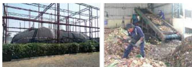
Figure 6: Bio-CNG Plant site, Kabitkhedi Plant
