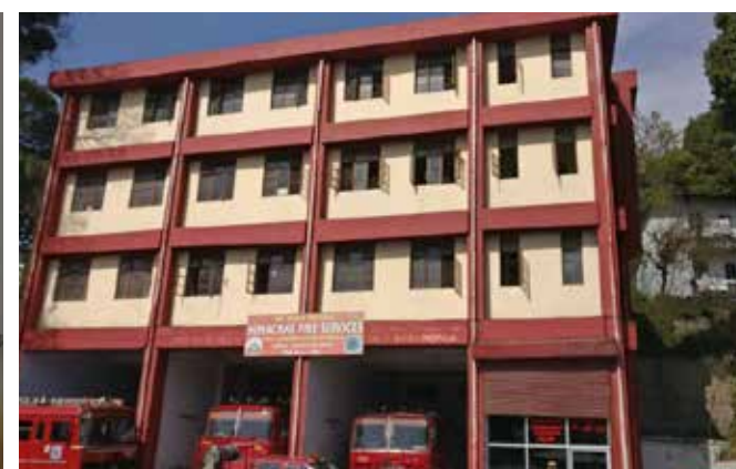
Figure-9: Fire station with trees on both sides creating shadows Source: Rooftop Solar detailed project report
