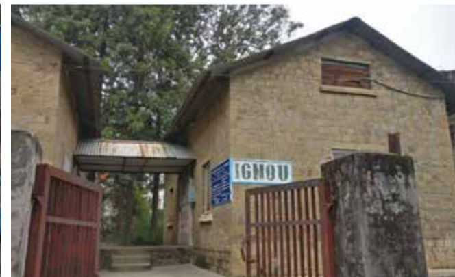
Figure-12: IGNOU building with small roof area and inappropriate orientation Source: Rooftop Solar detailed project report
