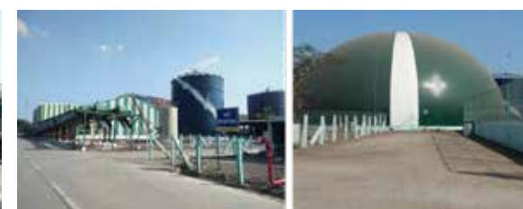
Figure 7: Bio-CNG Plant site, Devguradiya Plant
