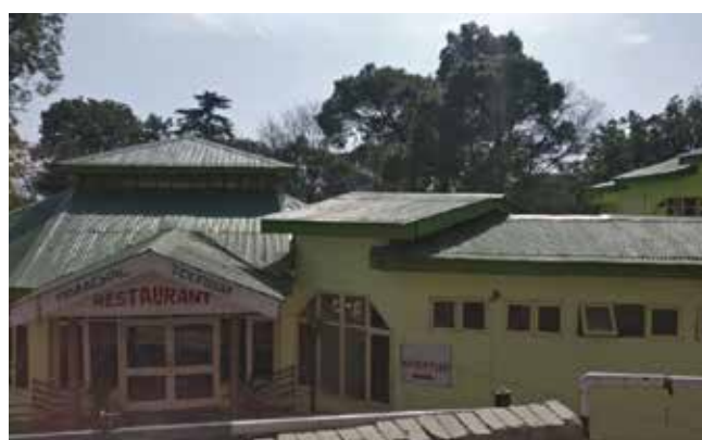
Figure-10: Inclined roof of hotel Kunal with trees in the rear Source: Rooftop Solar detailed project report
