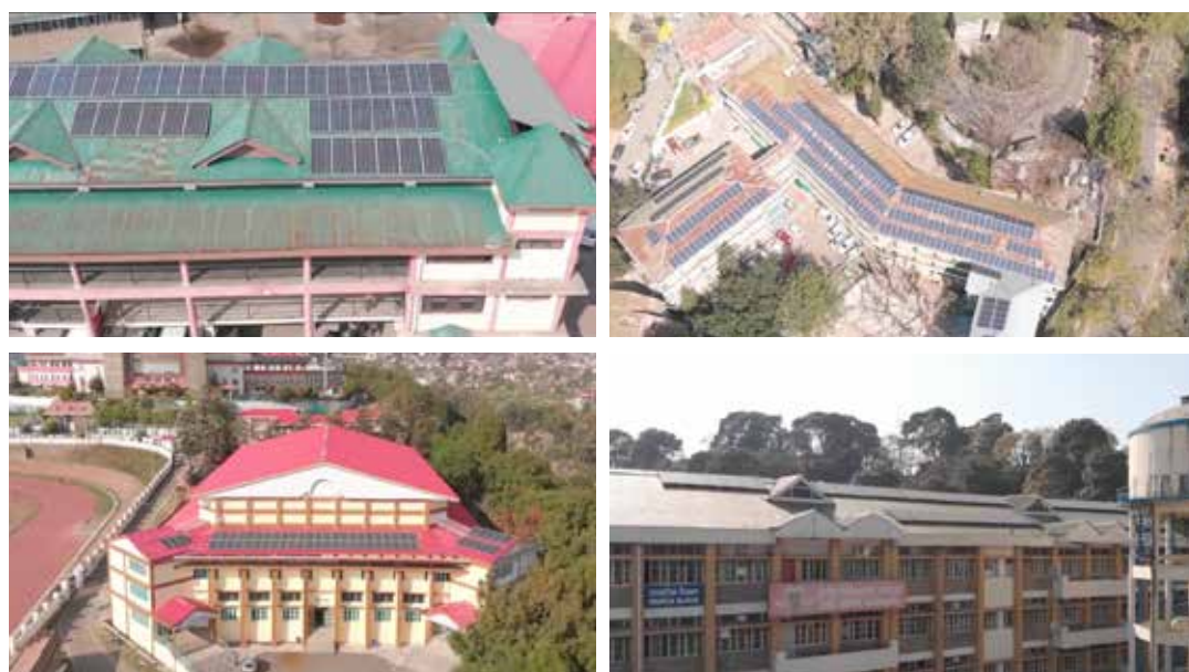
Figure 13. Solar PV system installed on buildings in phase I Source: Dharamshala Smart CitySource: Rooftop Solar detailed project report
