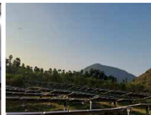
Plate 8. Land based smart solar panels that change directions as per sun path, maintained by GVSCCL
