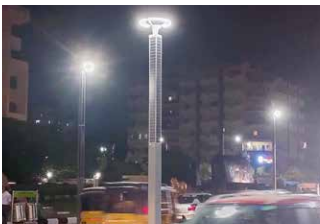
Plate 13. Smart Solar Street Lights at Beach Road, Visakhapatnam
