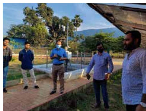
Plate 6. SPAV Team inspecting GVMC maintained land based solar panels
