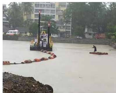
Figure 9 The dredging and desilting process (Source: Mangalore Smart City Limited)
