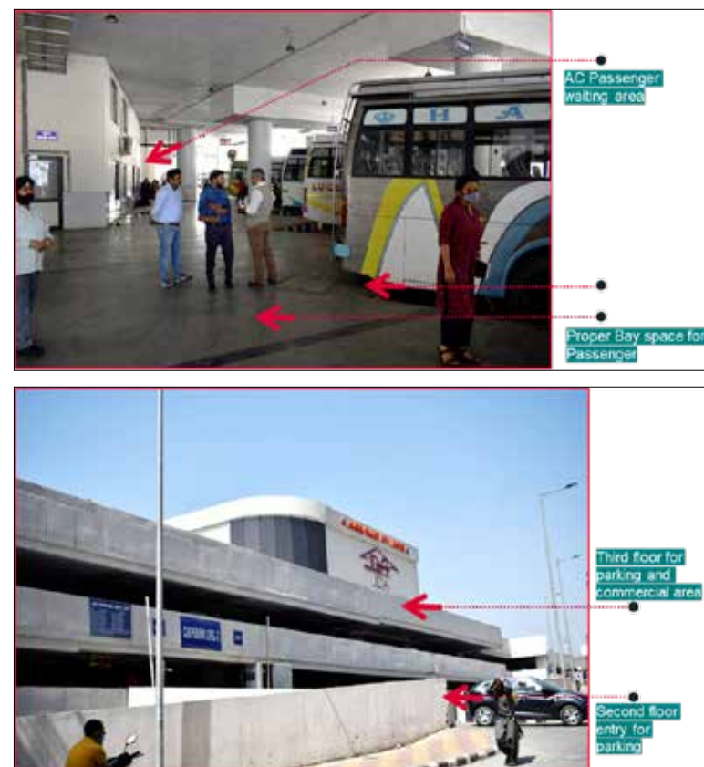
Figure 3.6: Bus stand facility
