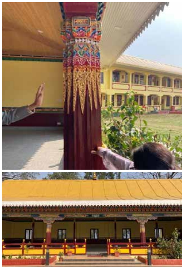
Figure 14: One of the older columns in the Yabring restored (L), the restored Yabring (R)
