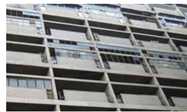
Figure 2.5: Encroachments covering the original veranda Source: Chandigarh Heritage Report by Heritage Conservation Committee of Chandigarh
