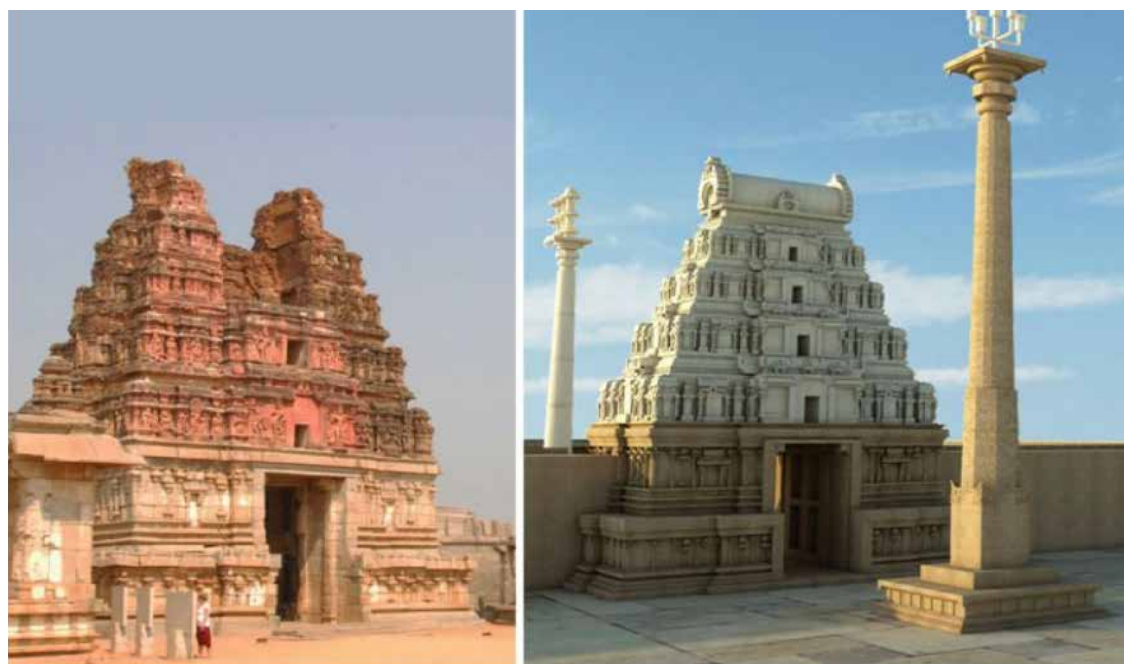
Figure 2: Reconstruction of deteriorated structure through texture mapping.; Source: Mallik, A, Chaudhury, S, Chandru, V, & Srinivasan, S 2017. Digital Hampi: Preserving Indian Cultural Heritage
