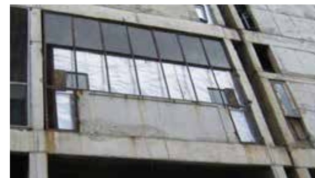
Figure 2.6: Extension in the original veranda Source: Chandigarh Heritage Report by Heritage Conservation Committee of Chandigarh
