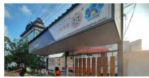
Figure 3: Smart Bus shelter
