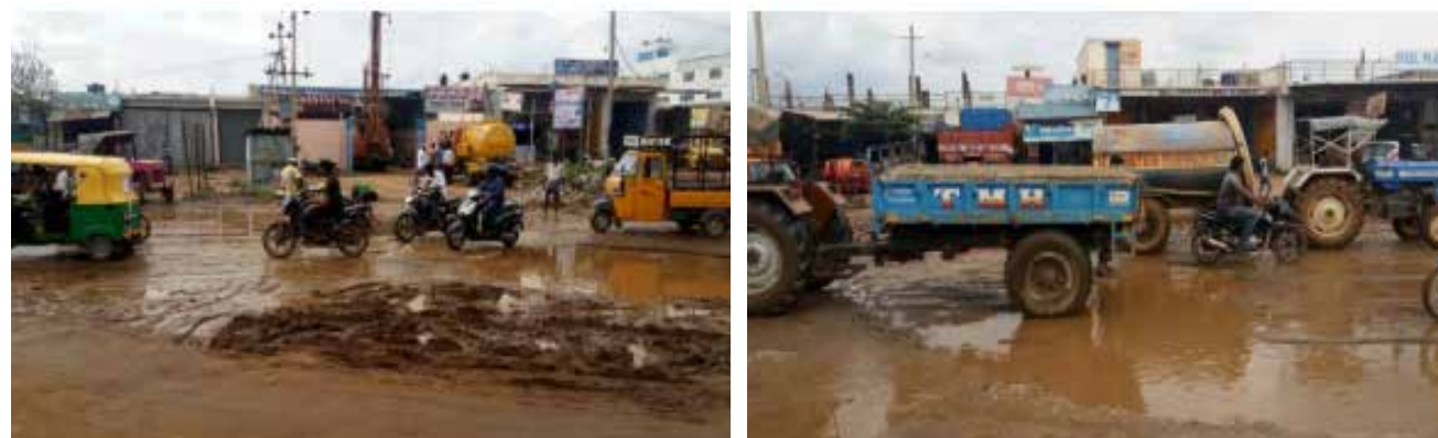
Figure 02: Pre-existing condition of the Ring Road, Source: Detailed Project Report
