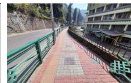
Figure 2: Improved footpath at Zero Point, Baluwakhani
