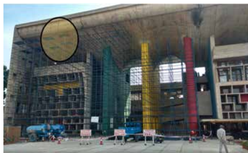
Figure 2.18: Image of High Court before restoration Source: CSCL
