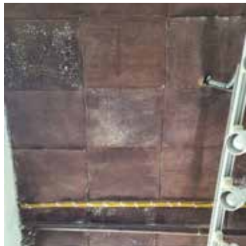
Figure 2.32: Final restored ceiling Source: Ar. Deepika Gandhi
