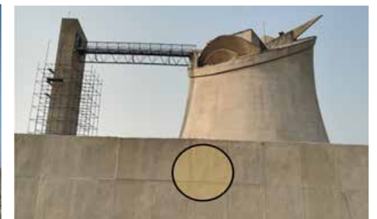
Figure 2.21: Image of the Secretariat after restoration Source: CSCL
