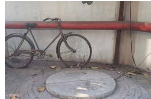
Image 8: Percolating recharge well
