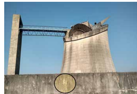
Figure 2.20: Image of the Secretariat before restoration Source: CSCL
