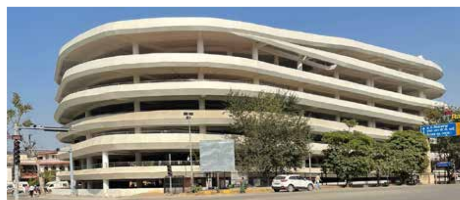
Figure 7: View of Collectorate Multilevel Parking Source: By author
