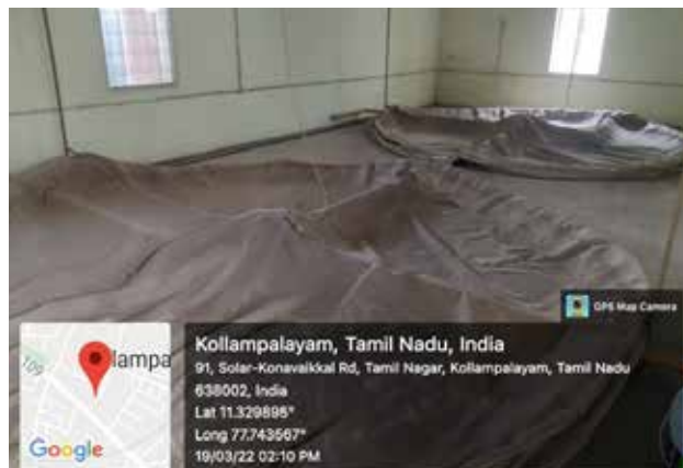
Figure 15. Methane gas balloons Source: Author
