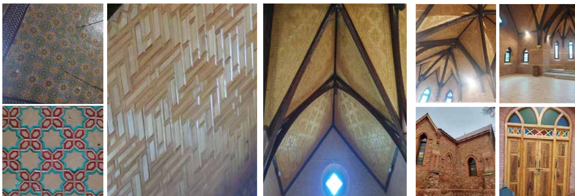
Figure 3: Clockwise from top a. Pattern of Khatamband ceiling in Khankah-e-Maula, Srinagar, b. pattern of restored Khatamband ceiling St. Luke's Church c. restored Khatamband ceiling and roof truss St. Luke's Church. d. Pattern of Khatamband walls in Ziyarat Naqashband Sahab Source: author
