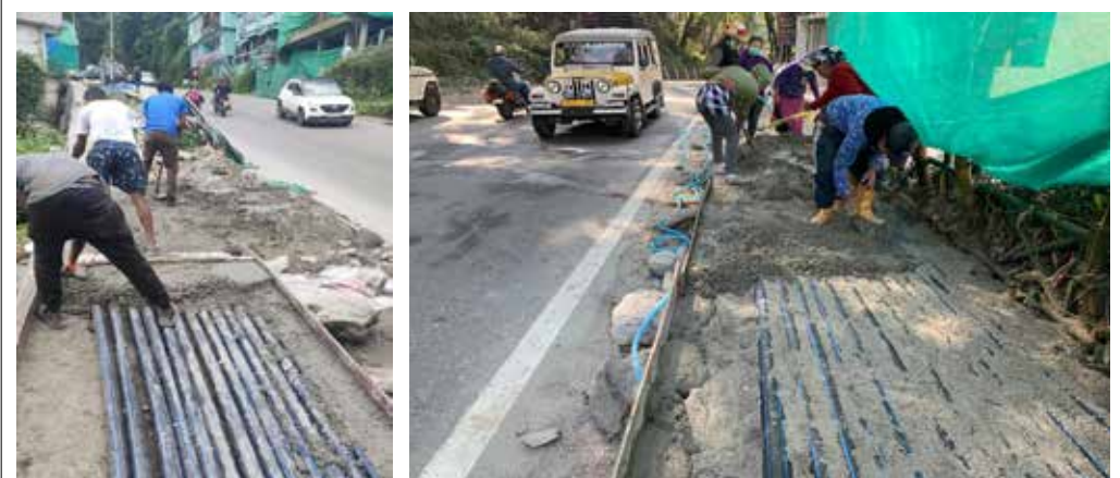
Figure 10: Laying of HDPE pipes Source: GSCDL
