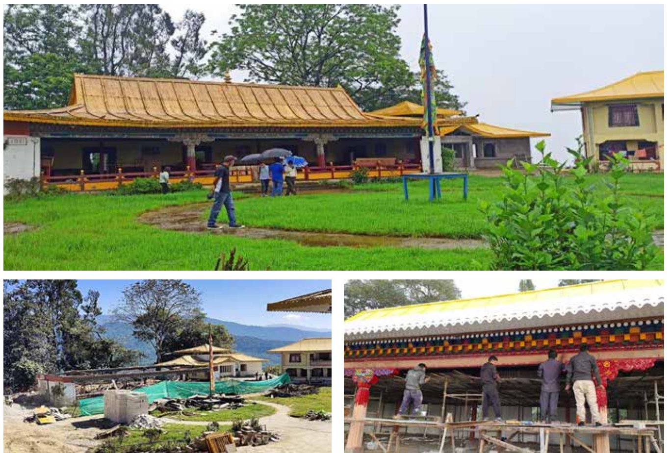
Figure 15: (Clockwise from top left) The Yabring in dilapidated state, Removal of the walls of the Yabring, Painting works by 'Laripa'
