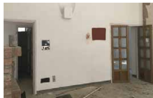
Figure 2.27: The final restored light niche; Source: Author
