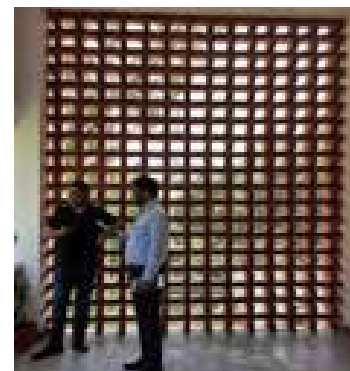
Figure 2.30: The final restored jaali, Source: Author
