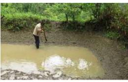
Using a pole tied to a gunny bag, a farmer rams and compresses the side wall of a pond
