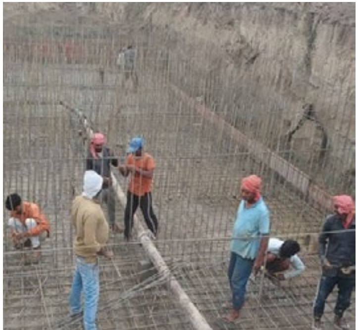
Construction of FSTP in Rudrapur
