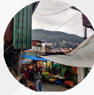
Tangled electric wires
