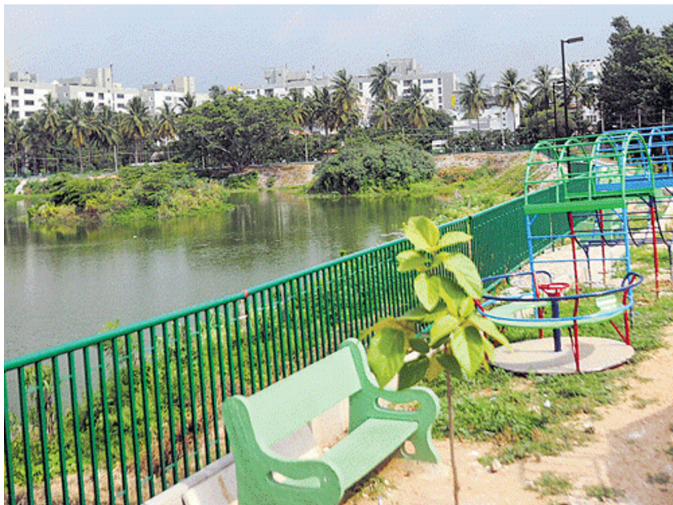
Figure 7: Example of cast iron railing fencing for boundary protection of water bodies
