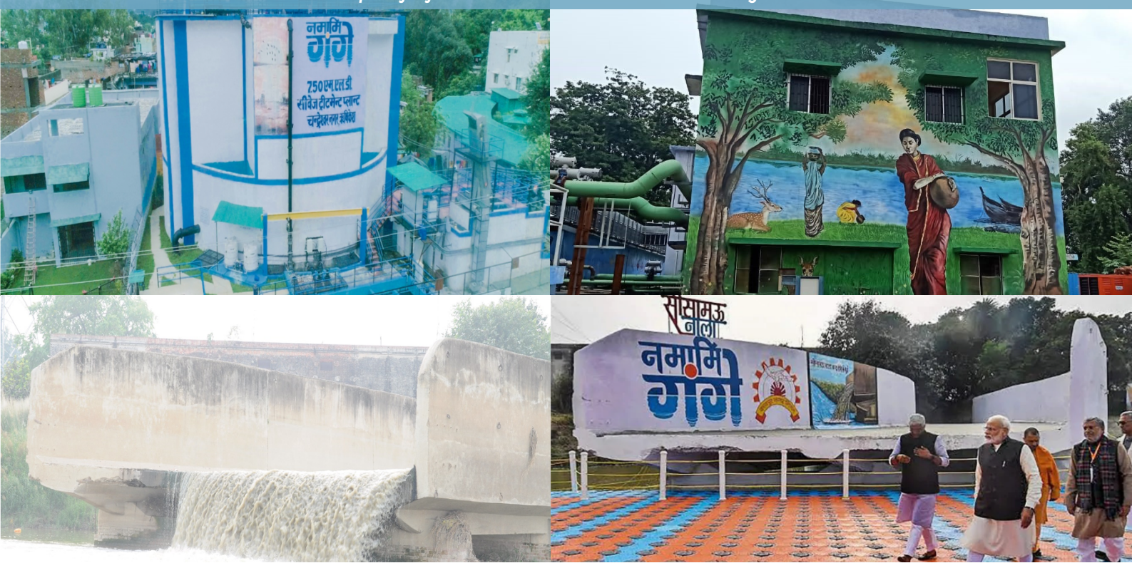
Glimpse of infrastructure created under Namami Gange Mission
