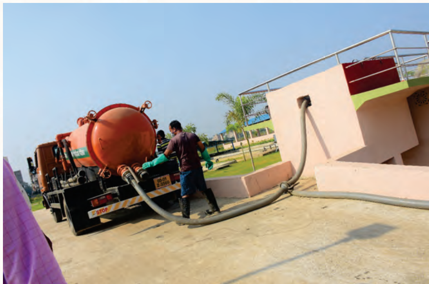
Faecal Sludge and Septage Management (FSSM) Plant at Basuaghai
