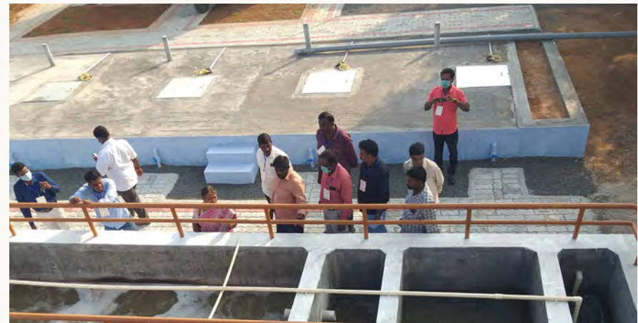
Storage Tank (Collection Tank)
