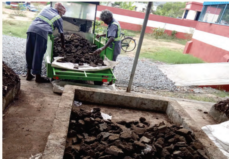
Dried sludge from the sludge drying beds is collected and transported to Resource Recovery Park for further treatment
