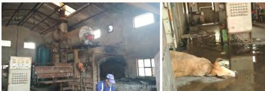
Animal Carcass Incineration Plant
