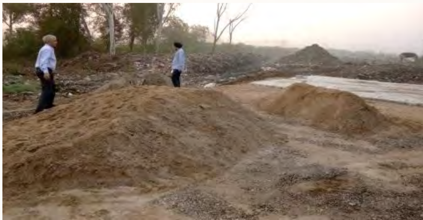
Remediation of the existing dumpsite
