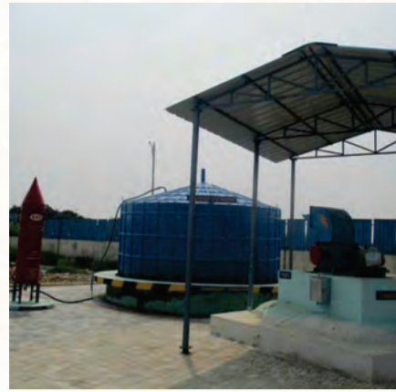
50 cubic meter Biomethanation Plant
