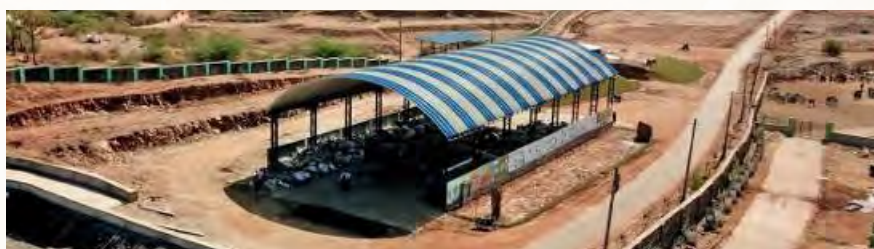
Material Recovery Facility (MRF) Unit
