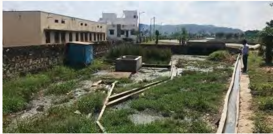
Drain Water Treatment Plant
