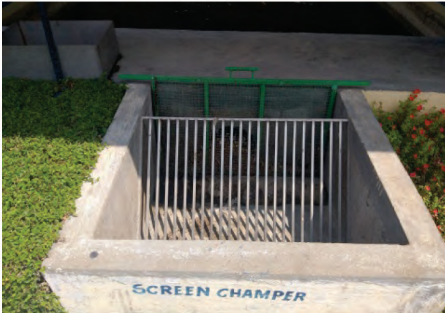
Screened Inlet Chamber
