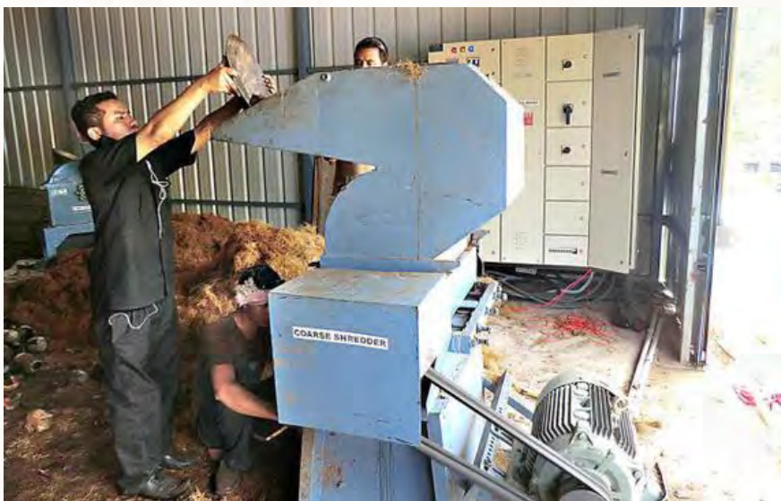
Shredding of Cocount at Coconut Waste Processing Plant
