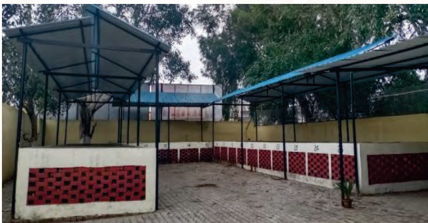
NADEP Composting pits at SWM Plant
