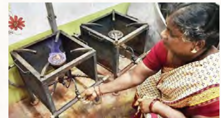
The gas produced being used in the Kitchen
