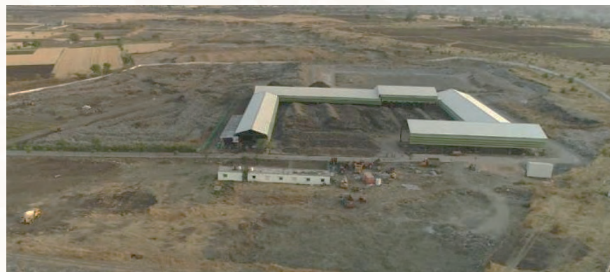
Preparatory section unit of compost plant
