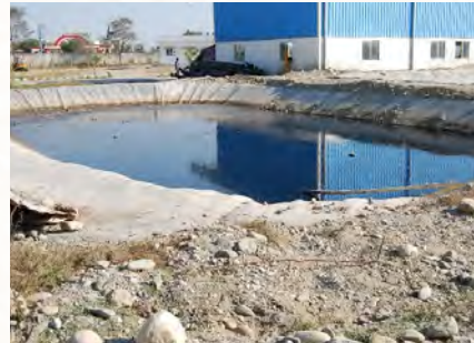
Solar Evaporation Pond
