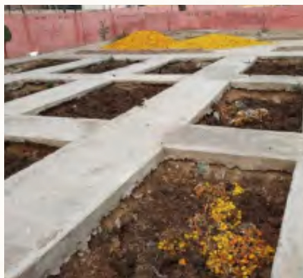
Composting pits at the facility
