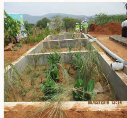
Septage from Feeding Tank is led into Vertical-flow Constructed Wetland
