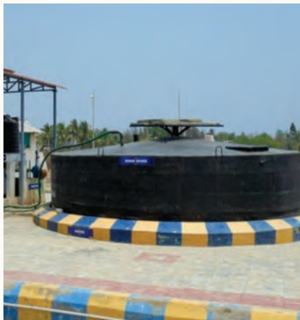
50 cubic meter Biomethanation Plant
