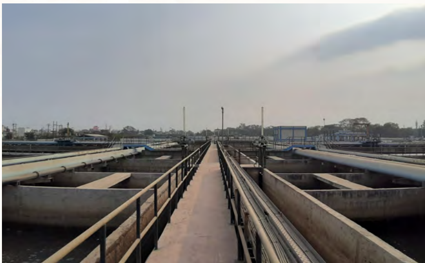
Sequencing Batch Reactors (SBR) based STP
