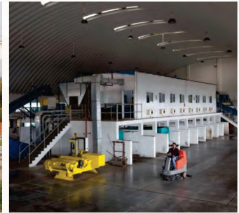
Sorting Station with bunkers to sort 15 fractions
