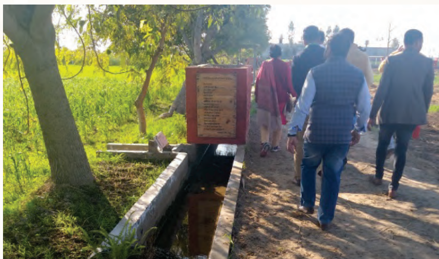
Irrigation canal connecting with the rainwater harvesting tank and the NADEP Composting Pit
