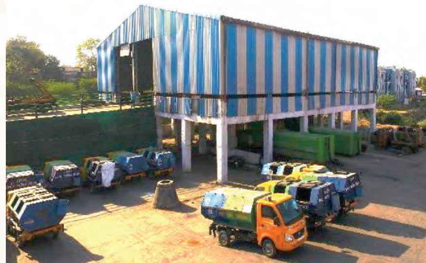
Waste Transfer station
