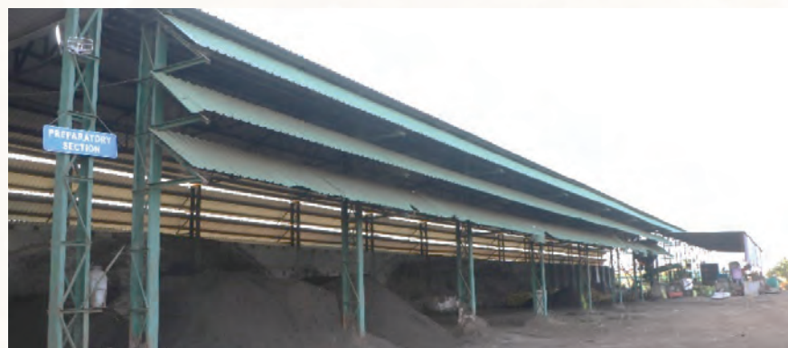
Preparatory section unit of compost plant
