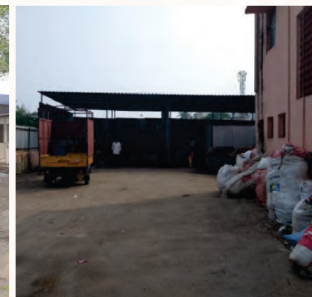
Dry waste shed at ward level
