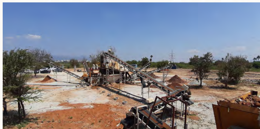
Construction and Demolition Plant at Thukivakam
