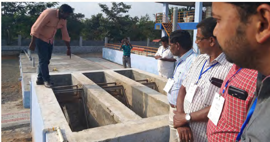
Septage Receiving Station
