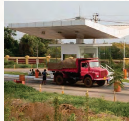
Weigh Bridge Station
