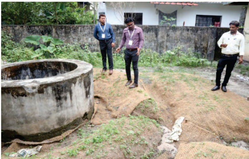
Well recharging at the office complex
