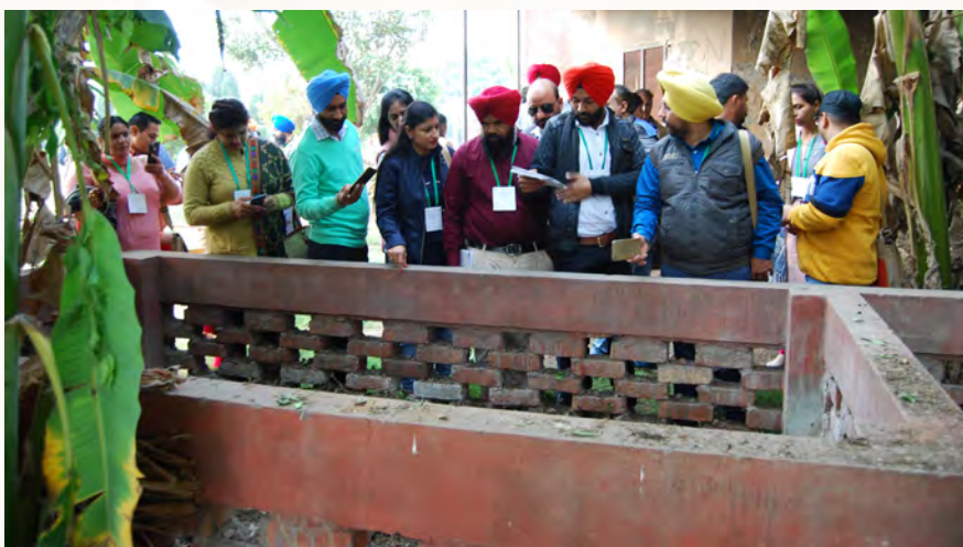
Decentralised Composting Units at Schools in Nawanshahr
