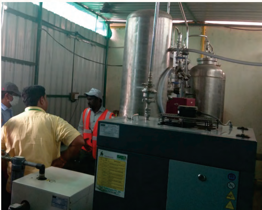
Biogas stored in the biogas holder
