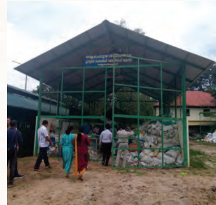
Resource recovery facility
