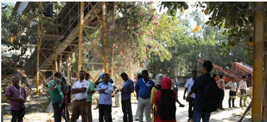
Construction and Demolition Waste Management plant at Chikkajala
