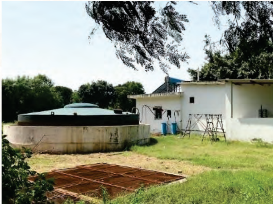
Bio-Methanation-Cum Electricity Generation Plant
