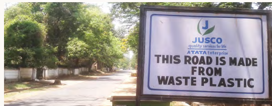
Road is made from waste plastic
