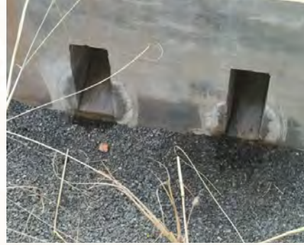
Treated water from Horizontal-flow Constructed Wetland sent to collection tank
