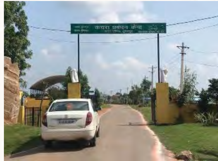
Integrated Solid Waste Management facility
