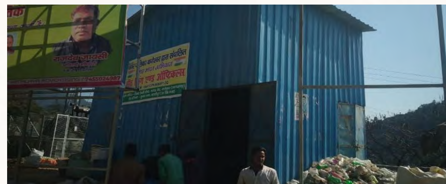
Material Recovery Facility at Garur Road, Bageshwar
