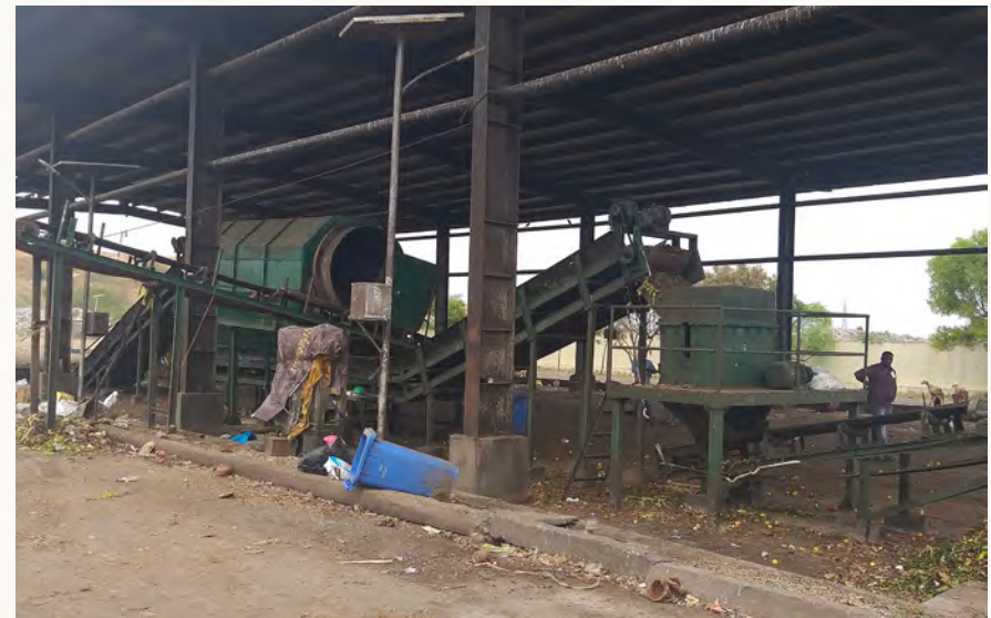
Incoming wet waste is sorted and shredded
