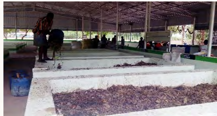
Composting pits at the facility
