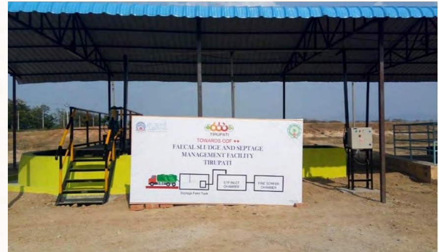
Faecal Sludge Treatment Plant (FSTP) at Thukivakam
