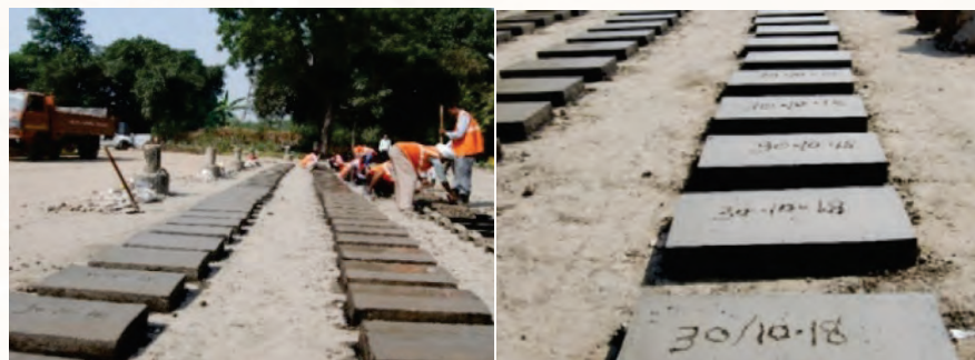
Concrete mix is poured into the frames and left to set
