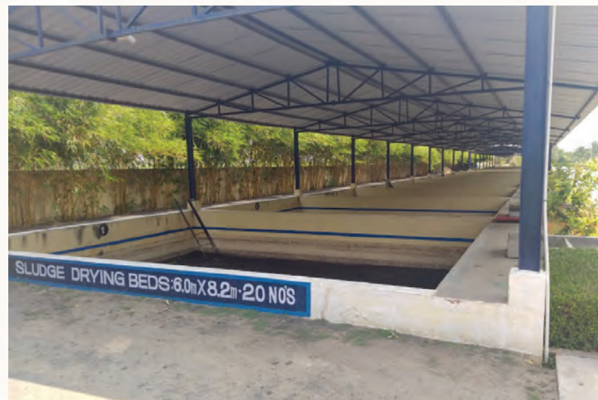
Sludge drying bed
