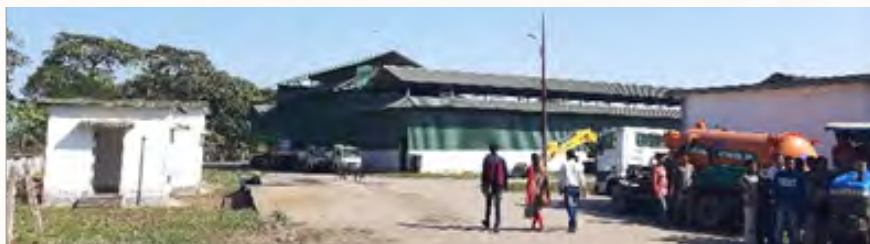
Integrated solid waste management facility
