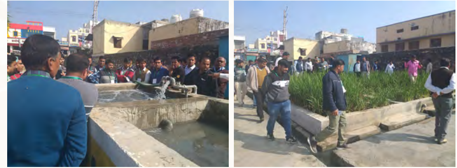
Treatment of Drainage water at the facility
