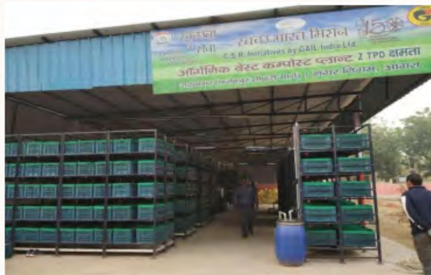
Organic Waste Compost Plant
