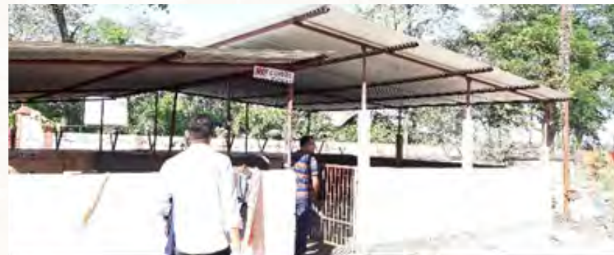
MRF (under Construction)
