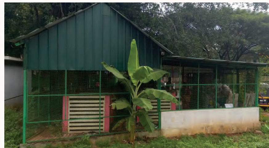
Waste Collection Centre
