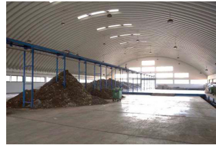
Figure 4.77: Fully enclosed compost shed
