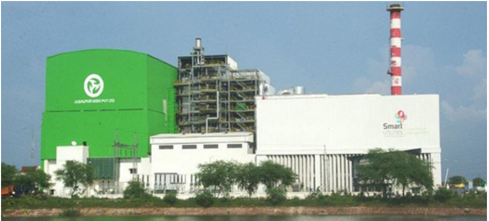
Figure 4.79: Jabalpur WtE plant
