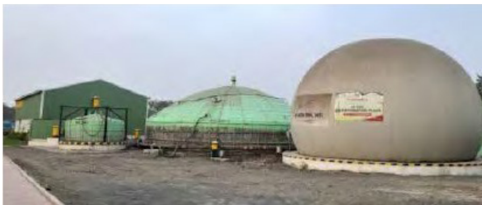
Figure 4.47: Main digester and balloon
