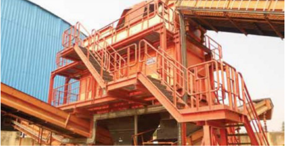
Figure 4.84: RDF facility by Ultra Tech, Jaipur
