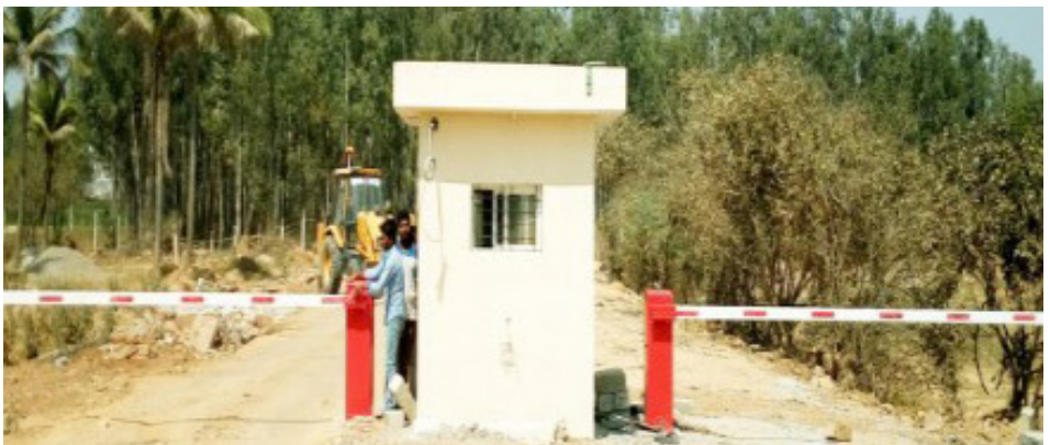
Figure 4.33: Vehicle scanner at entry point
