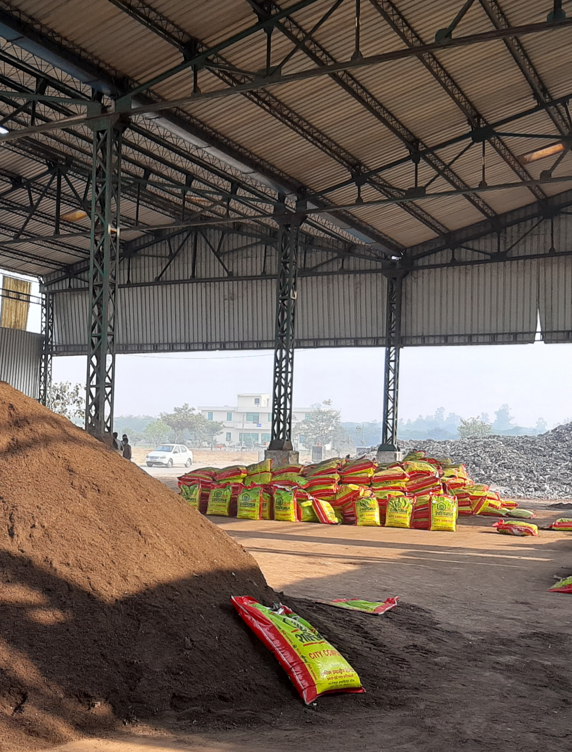
Compost packaging shed, Lucknow, Uttar Pradesh Source: Author
