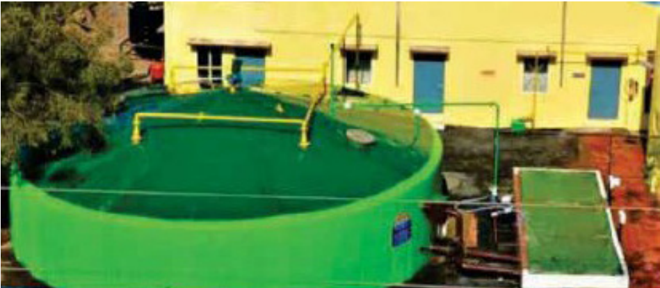
Figure 4.44: Biomethanation plant at vegetable market
