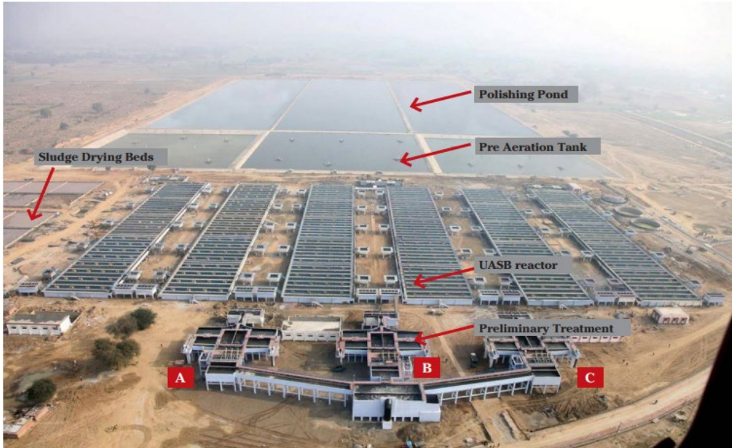
Figure 38: 345 MLD Lucknow UASB based STP along with Sludge Drying Bed
