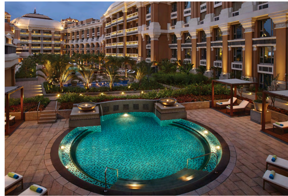
On the previous page: ITC Grand Chola Hotel - View of the courtyard.
