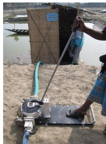
Source: Faecal Sludge Management System and Approaches
