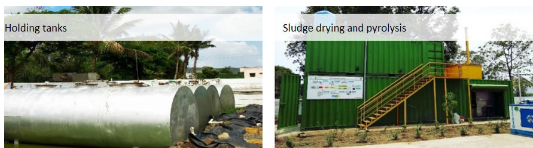
Figure 6 Site pictures of treatment plant
