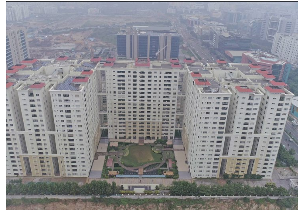
Abhra incorporating India's first district cooling systems for residential apartments
