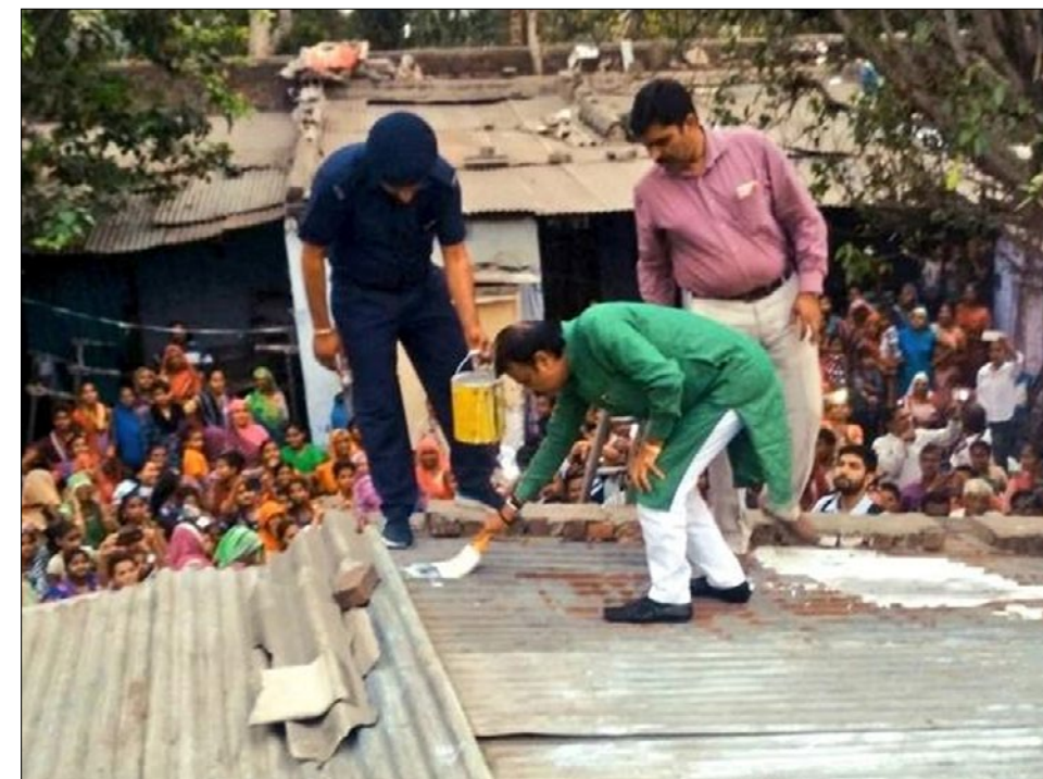
Training session on the application of the paint on the roof
