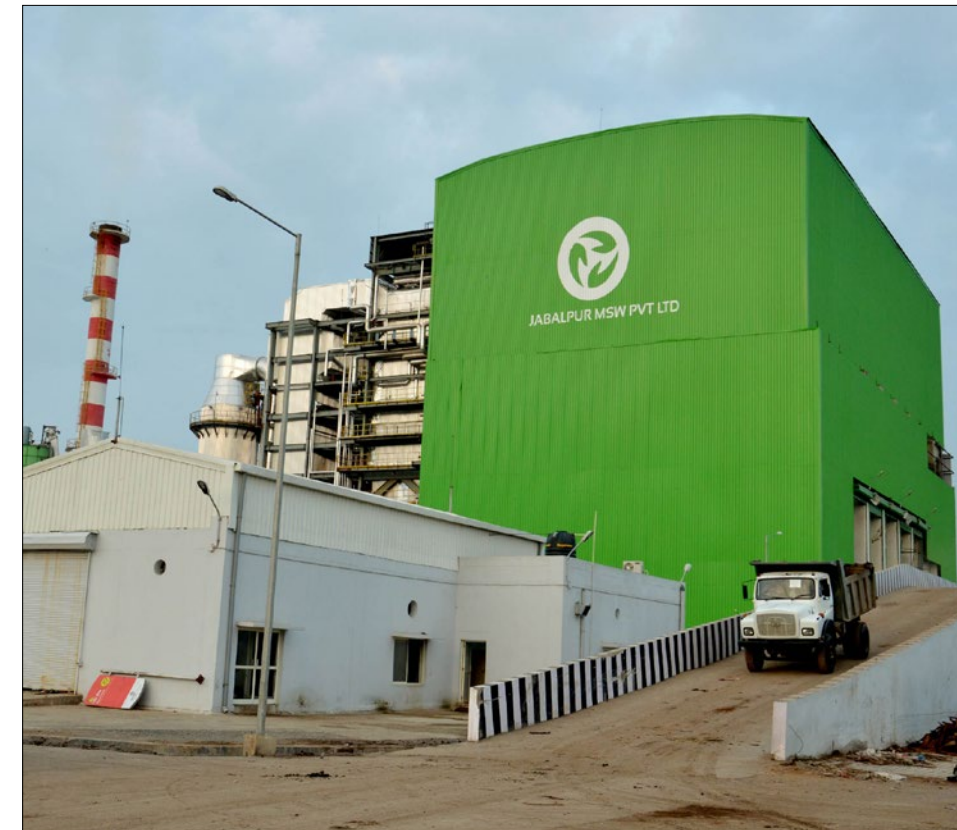
Waste management plant for the disposal of all kinds of municipal waste
