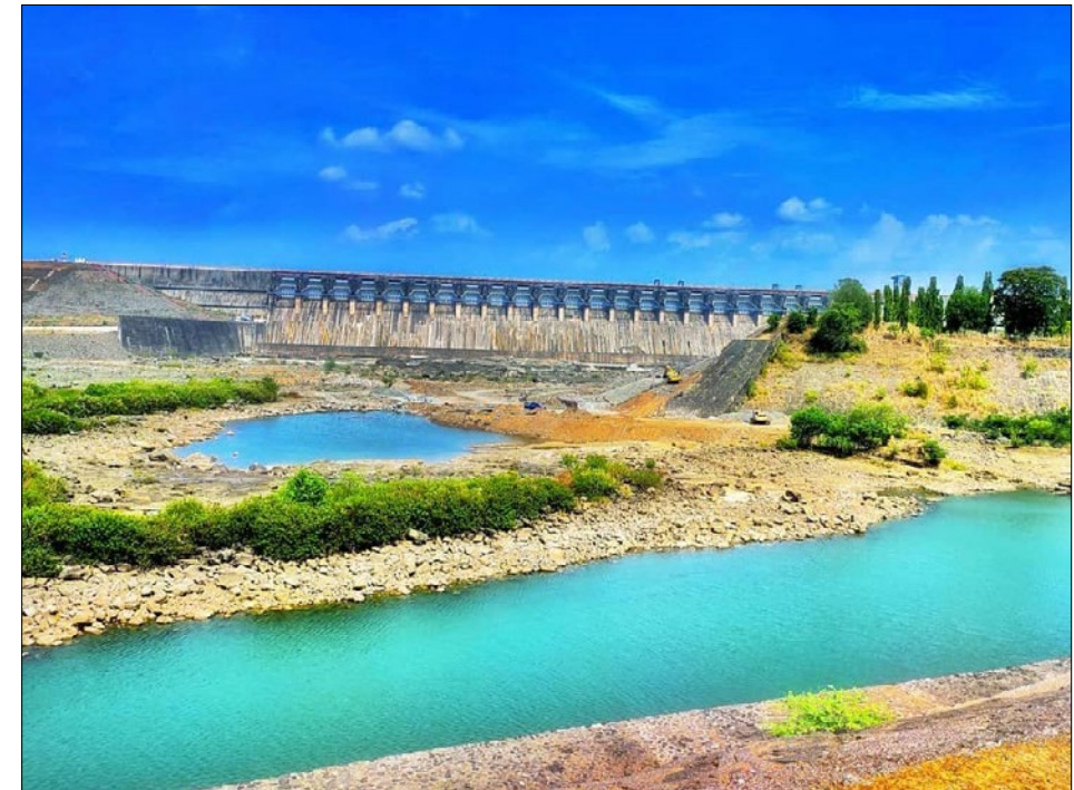
Ukai Dam has a catchment area of about 62,255 sq. km
