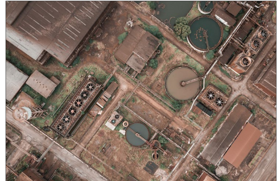
Sewage Treatment Plant addressing the need for sustainable water and sanitation
