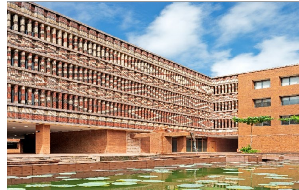
The built mass asserts a unique visual identity with a distinctive brick facade inspired by Ikat patterns
