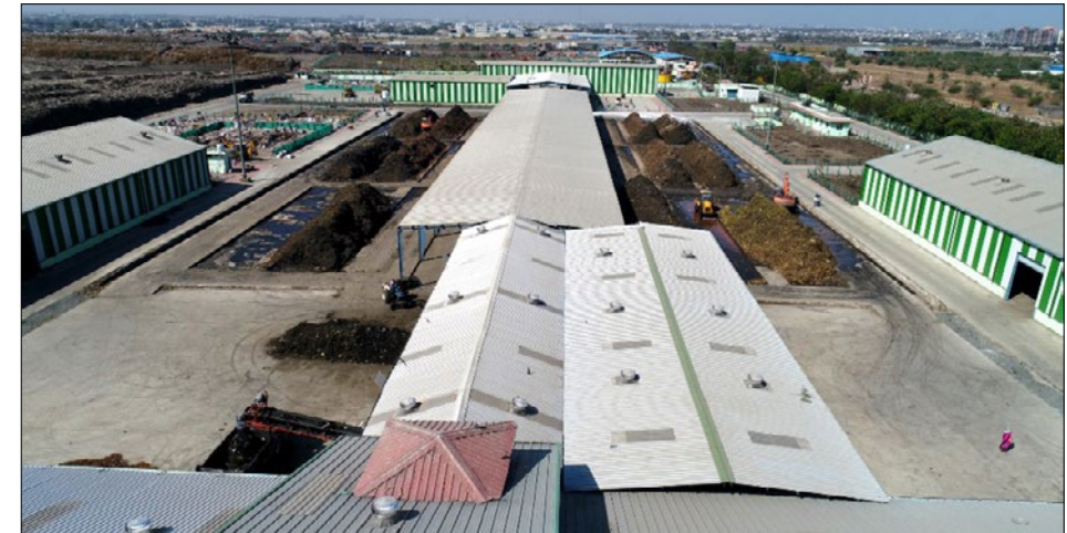
The processing and disposal site is around 146 acres
