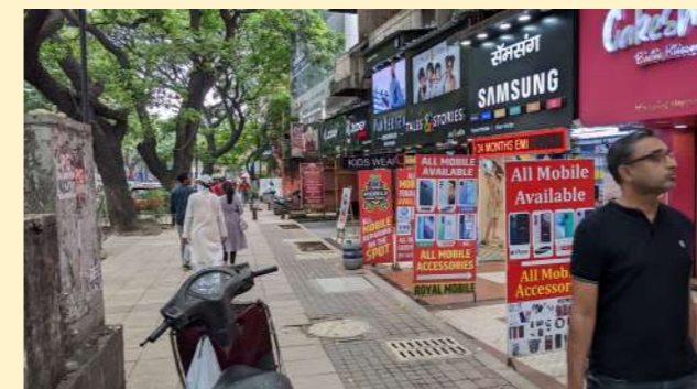
Fig. 83: Karve Road, Pune. Such streets have created welcome public spaces with high and active visitors' footfall, and have commercially viable frontages
