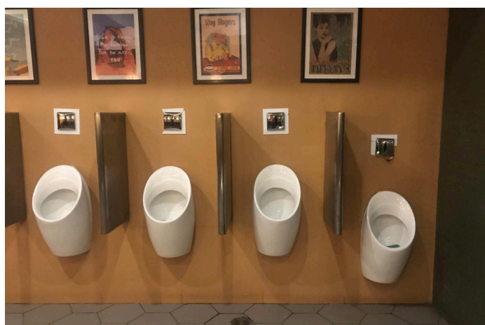
Image 5 Accessible and Child-friendly Wall-Hung Urinals Source: (Ministry of Housing and Urban Affairs, Government of India, 2021)
