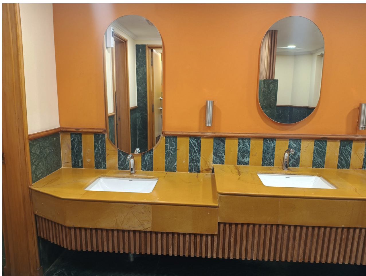
Image 10 Vanity-Top Accessible and Child-Friendly Wash Basins, India Habitat Centre, Delhi
