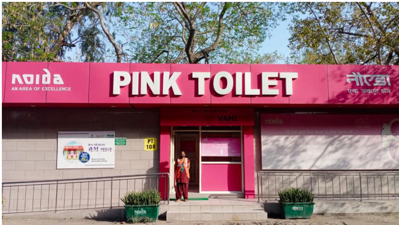
Image 2 Common accessible entrance facing the street, Noida Source: (Noida Authority, 2022)
