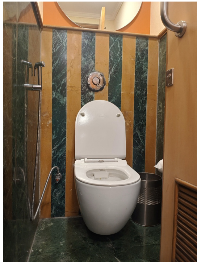
Image 8 Toilet Cubicle with Wall-Hung Western Water Closet, India Habitat Centre, Delhi Image Credits: Monica Thakur
