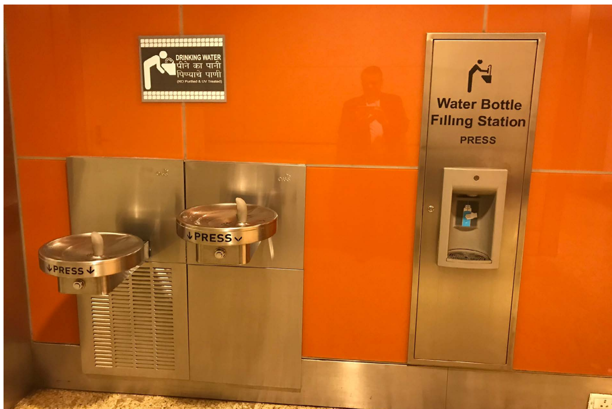
Image 5.10 Instructive signs at an accessible drinking water unit Photo Credits: Dr. Gaurav Raheja
