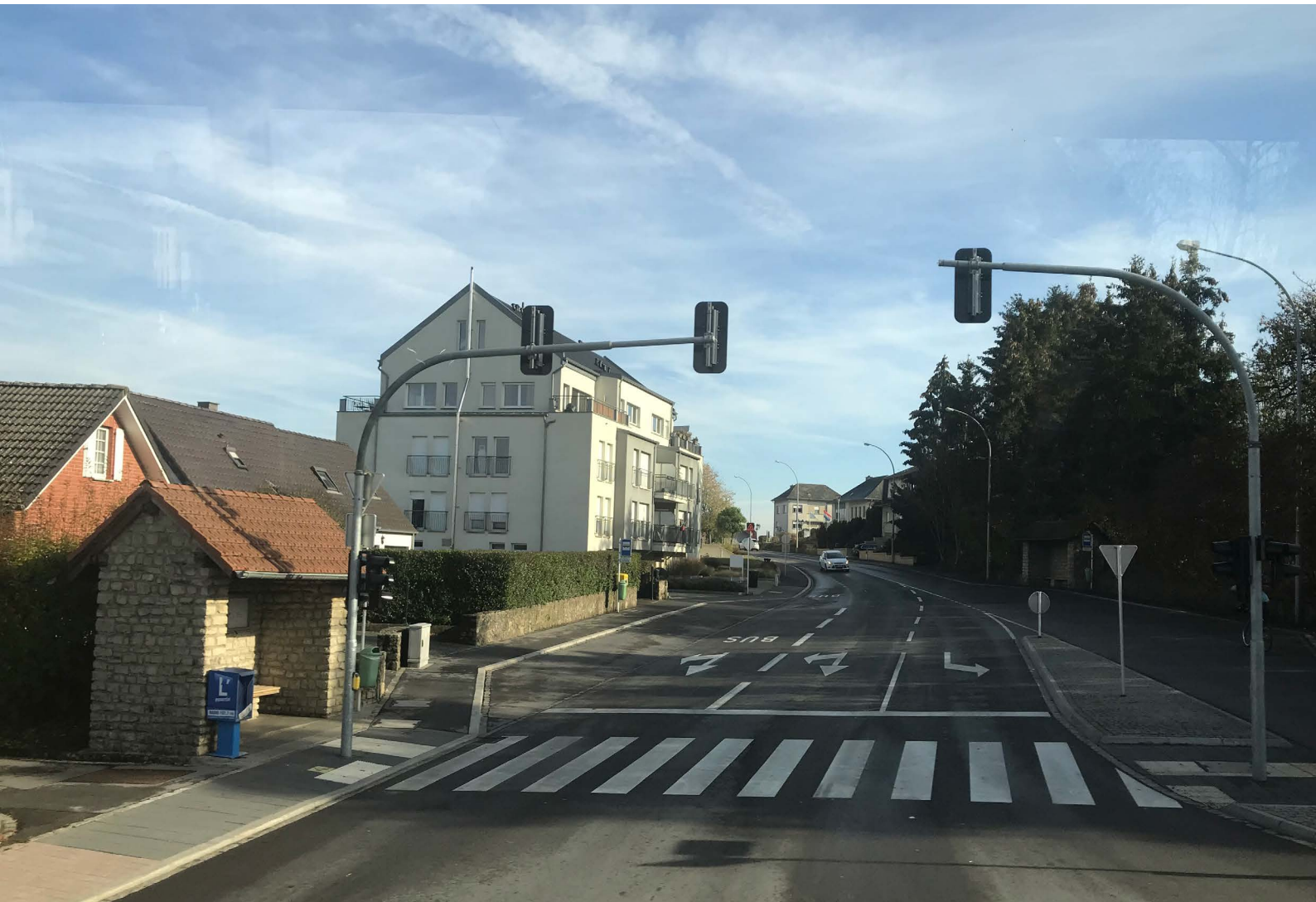
Image 3.15 Pedestrian crossing with pelican signals Photo Credits: Dr. Gaurav Raheja
