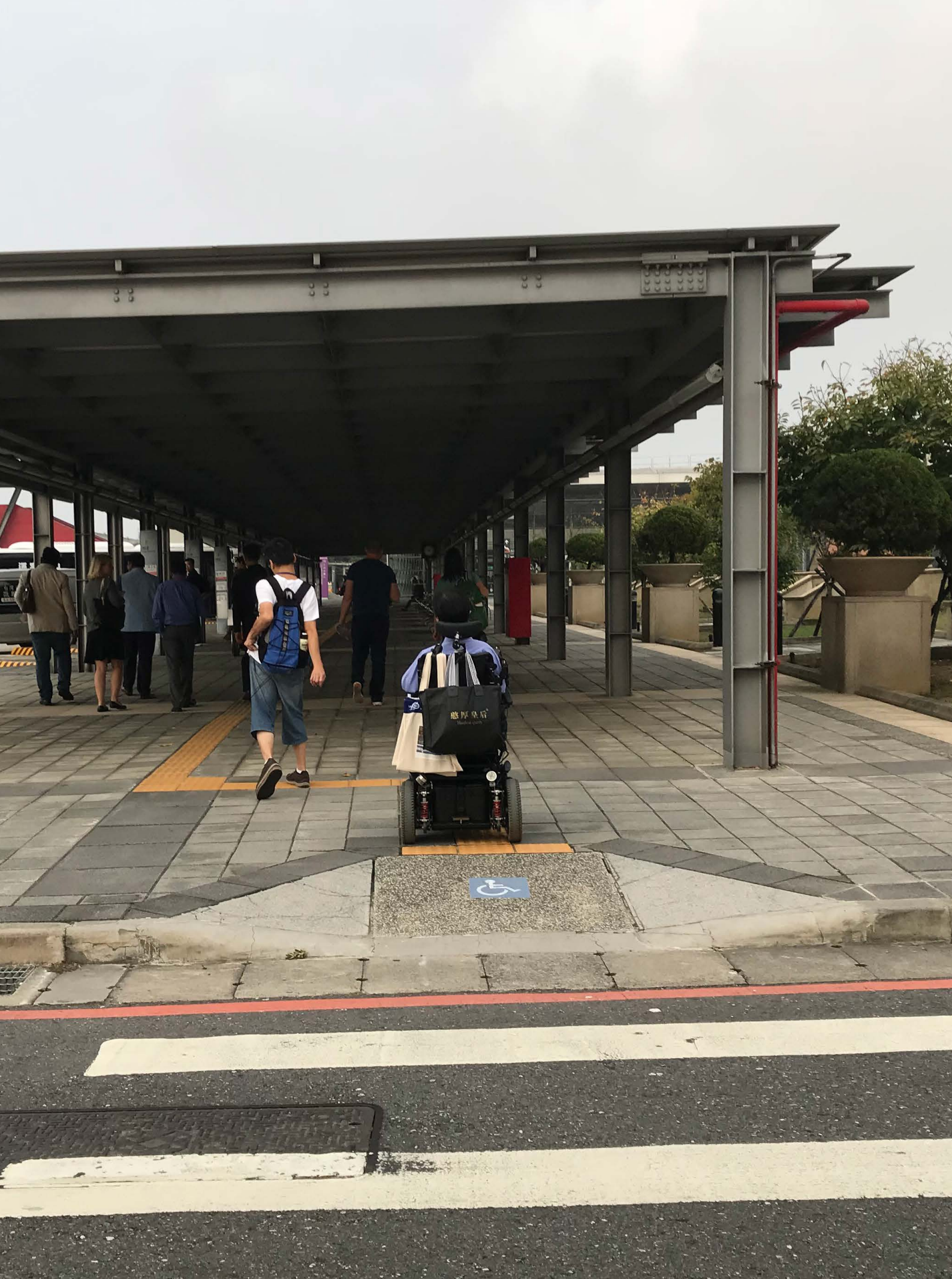
Image 3.13 Accessible flared kerb ramp at pedestrian crossing Photo Credits: Dr. Gaurav Raheja
