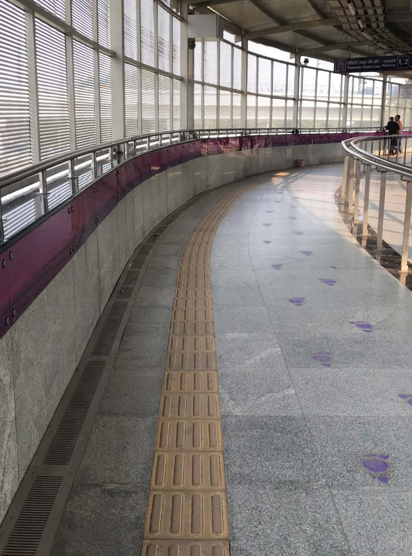
Image 3.21 Accessible horizontal circulation with handrail Photo Credits: Dr. Gaurav Raheja
