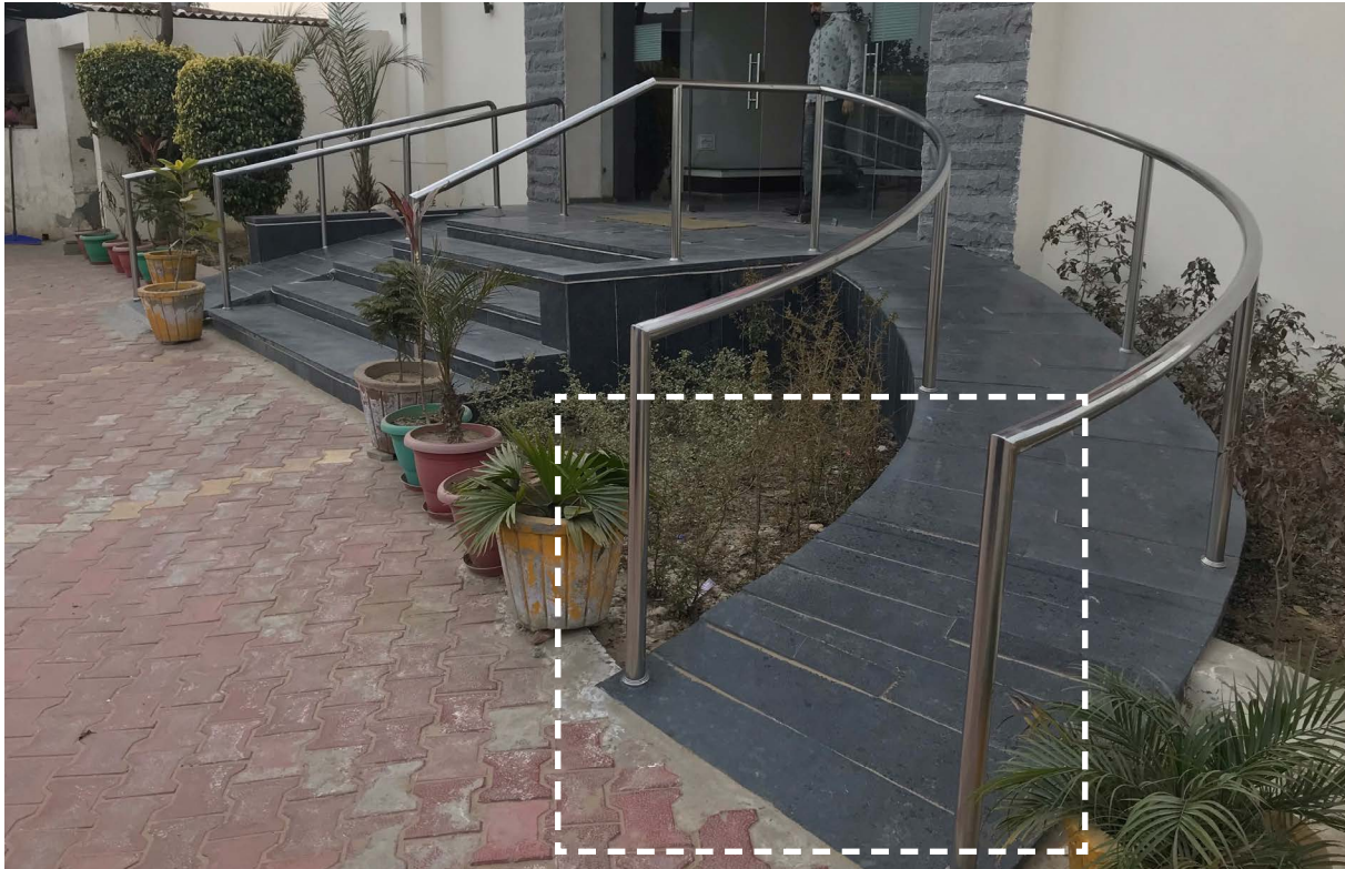
Image 2.9 Curved ramp with improper detailing and design
