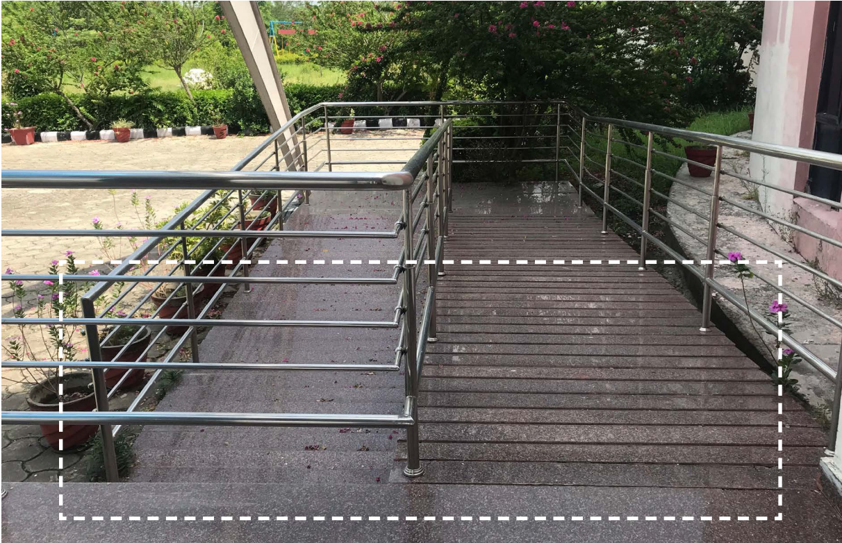
Image 2.8 Rumble granite strip on ramps as a barrier
