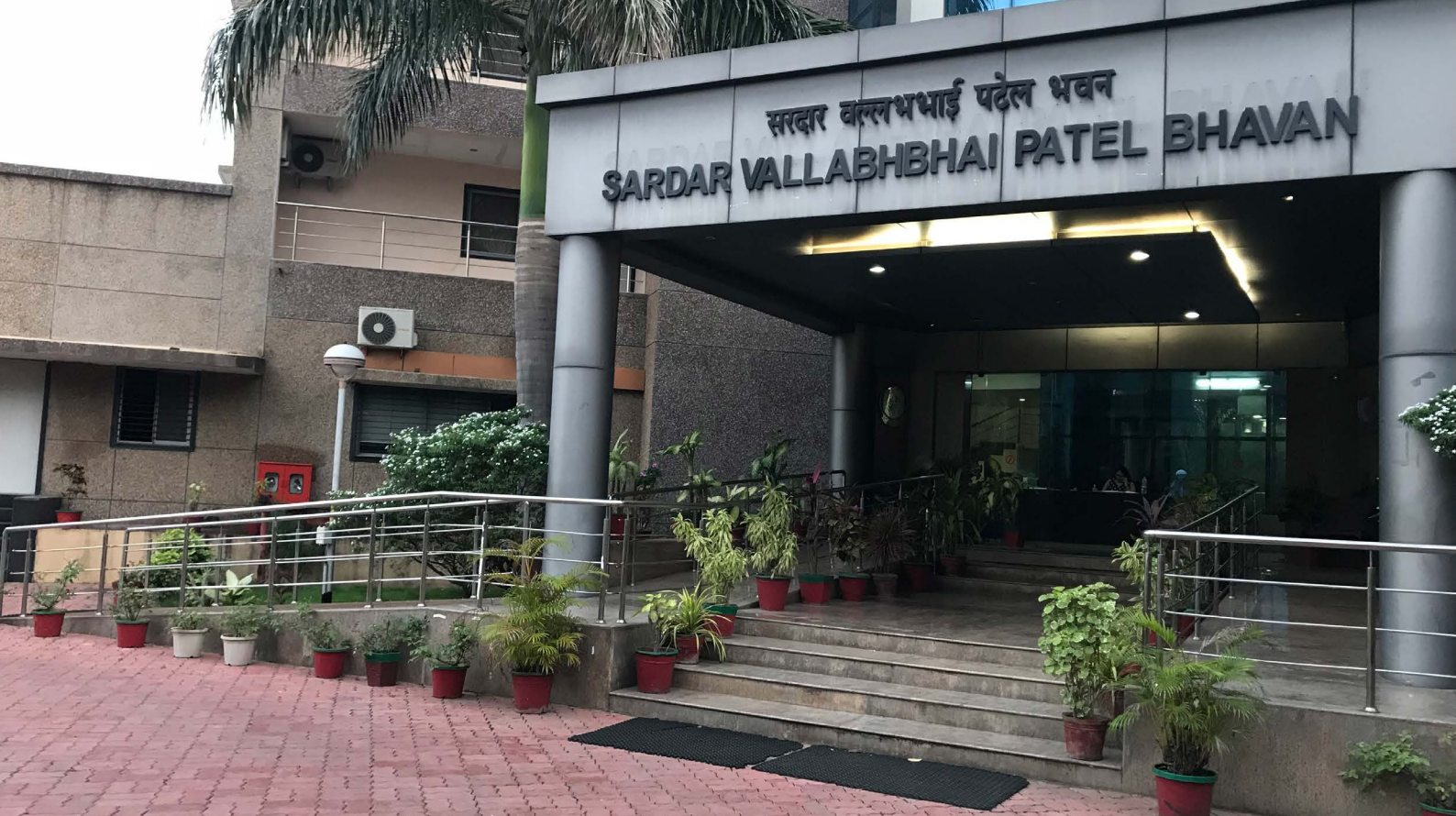
Image 6.35 Accessible entrance for office building Photo Credits: Dr. Gaurav Raheja
