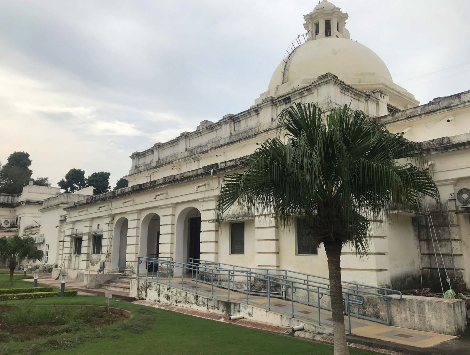
Image 7.7 Retrofitted accessible entrance through ramps in a heritage building Photo Credits: Dr. Gaurav Raheja
