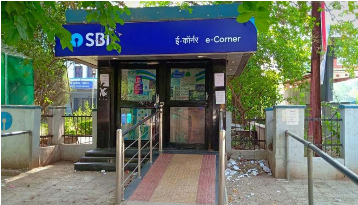
Image 6.58 Accessible entrance to a bank ATM
