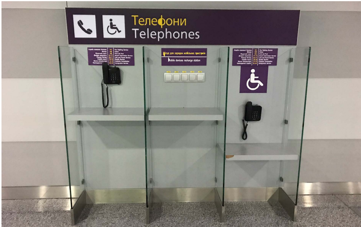
Image 5.9 Instructive signs at an accessible telephone unit Photo Credits: Dr. Gaurav Raheja
