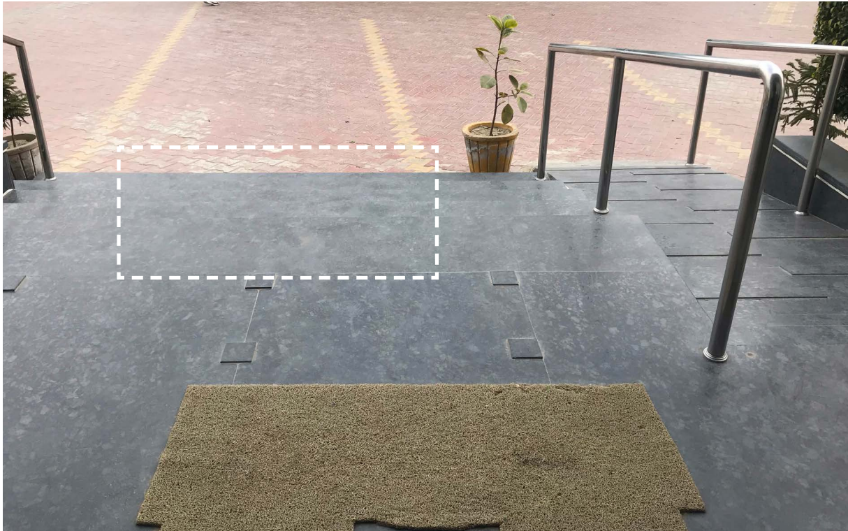
Image 2.18 Poor visual contrast in entrance steps
