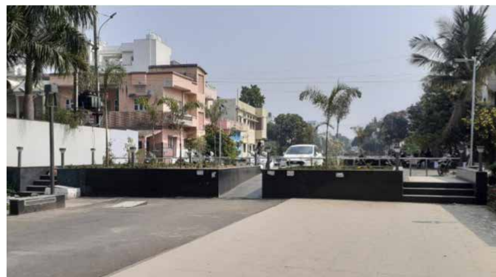
Figure 9: Entrance of the NMT corridor Source: Primary Survey
