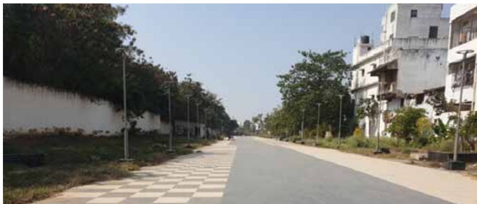
Figure 19: Showing the paving material on the track Source: Primary Survey
