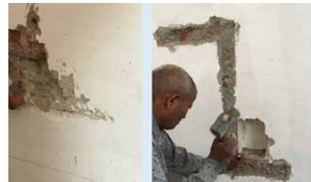
Figure 2.10: The niches being chiselled out of the wall Source: Ar. Deepika Gandhi
