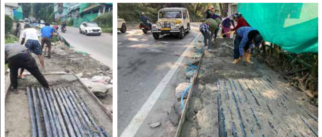
Figure 10: Laying of HDPE pipes Source: GSCDL
