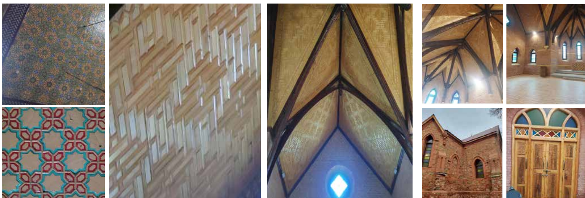
Figure 3: Clockwise from top a. Pattern of Khatamband ceiling in Khankah-e-Maula, Srinagar, b. pattern of restored Khatamband ceiling St. Luke's Church c. restored Khatamband ceiling and roof truss St. Luke's Church. d. Pattern of Khatamband walls in Ziyarat Naqashband Sahab Source: author
