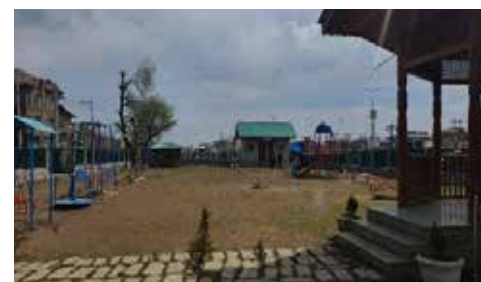
Figure 8: Various landscape elements like Gazebos, children play area with toilet facility and a coffee hut for revenue generation
