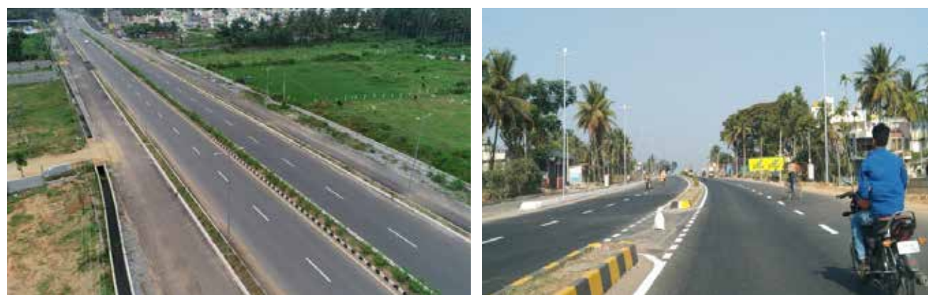
Figure 2: Pre-existing condition of the Ring Road Source: Detailed Project Report
