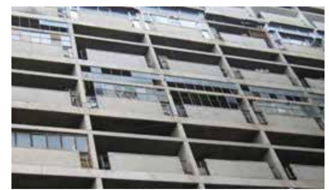
Figure 2.5: Encroachments covering the original veranda Source: Chandigarh Heritage Report by Heritage Conservation Committee of Chandigarh
