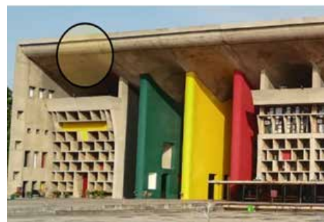
Figure 2.19: Image of High court after restoration
