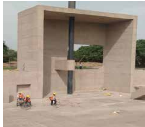
Figure 2.23: Image of the Open Hand monument after restoration Source: CSCL
