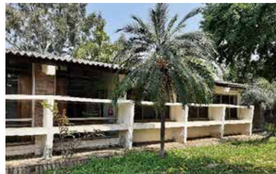
Figure 2.34 : Final restored louvres Source: Ar. Deepika Gandhi
