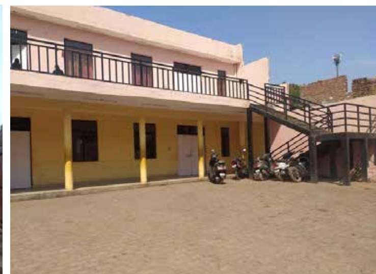
Figure 6: Micro Skill Development Centre at Kolhai in Tajganj. The ground floor is used for community activities, while the upper floor is being used for the training program.
