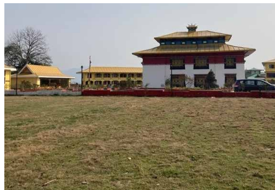
Figure 21: Excavated soil used at the site for levelling
