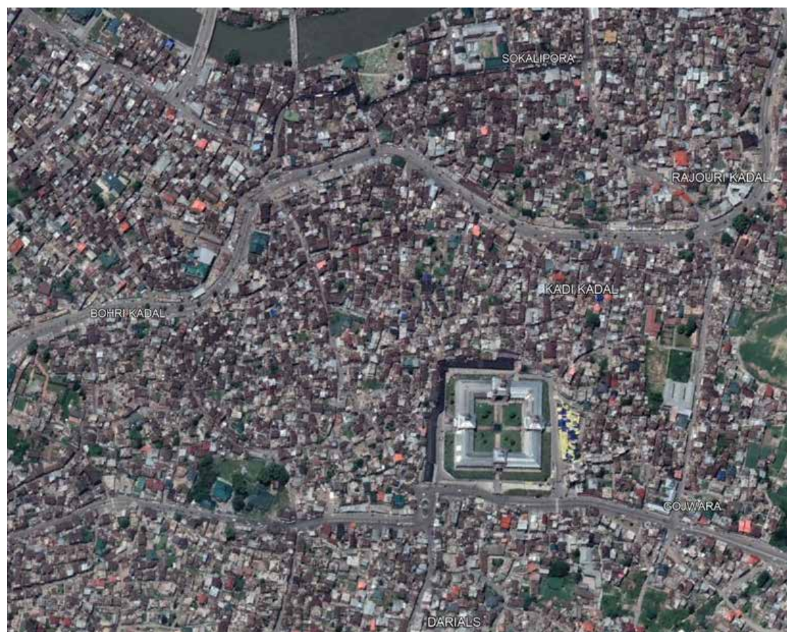
Figure 2. Satellite image of Jamia Masjid precinct, the mosque is located in a dense urban fabric surrounded by residential settlements all around. Source: Google Earth
