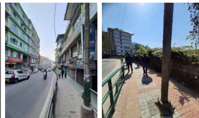
Figure 25: Street light poles blocking the footpath Source: IIT Kharagpur Survey
