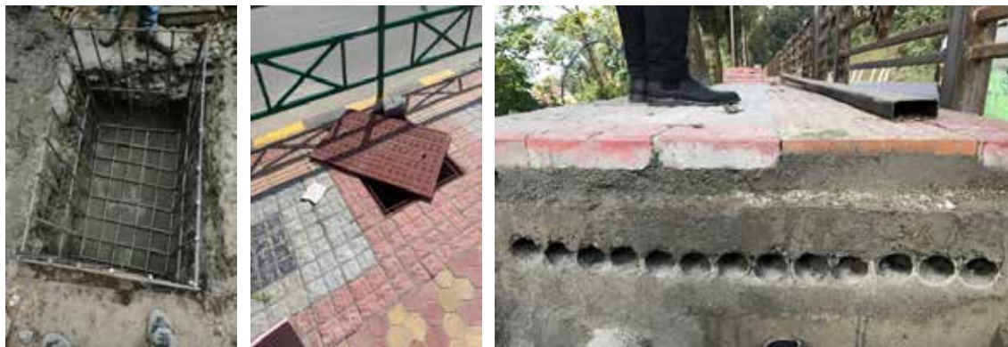
Figure 11: Manhole construction (left) & executed section with HDPE pipes (right) Source: GSCDL
