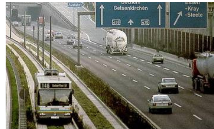
Montage of Guided busways in Essen, Germany
