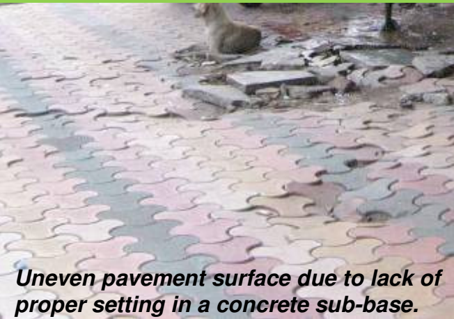
Obstructions that interrupt the walkway
