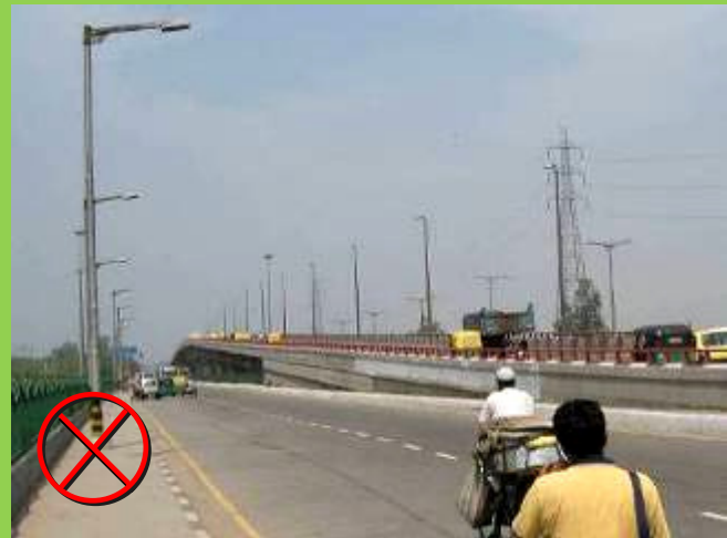
Light poles placed on the walkway so pedestrians are forced on to the road.
