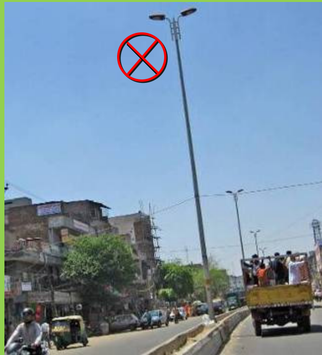
High Mast Lighting is inefficient and ineffective, especially in this narrow mixed-use street.
