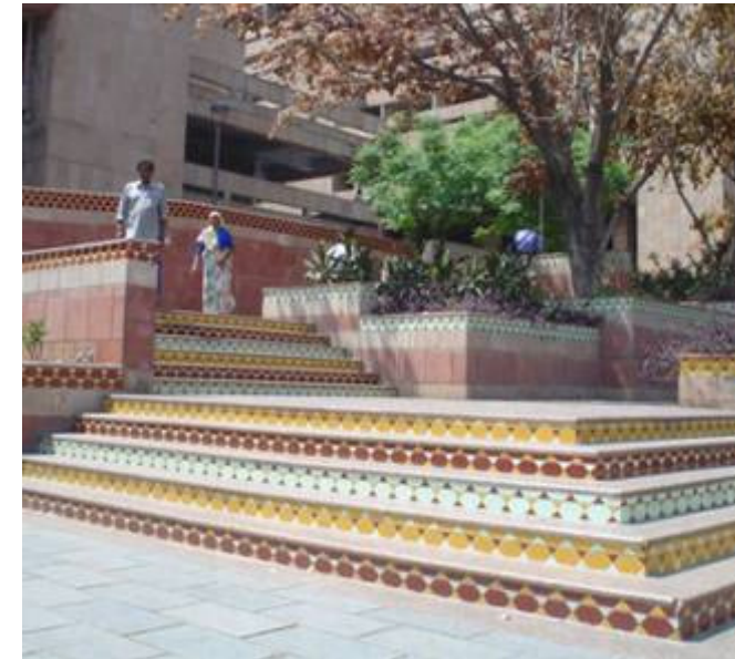
Ceramic Tiles use on vertical surfaces and risers of steps to add color (Bikaji Cama Place, Delhi)
