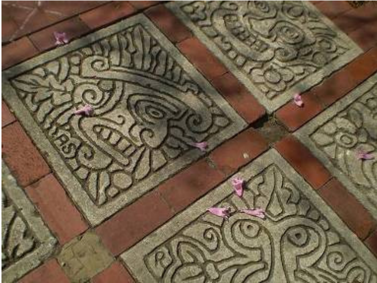
Public Art engraved Stone Tiles with brick tile paving.
