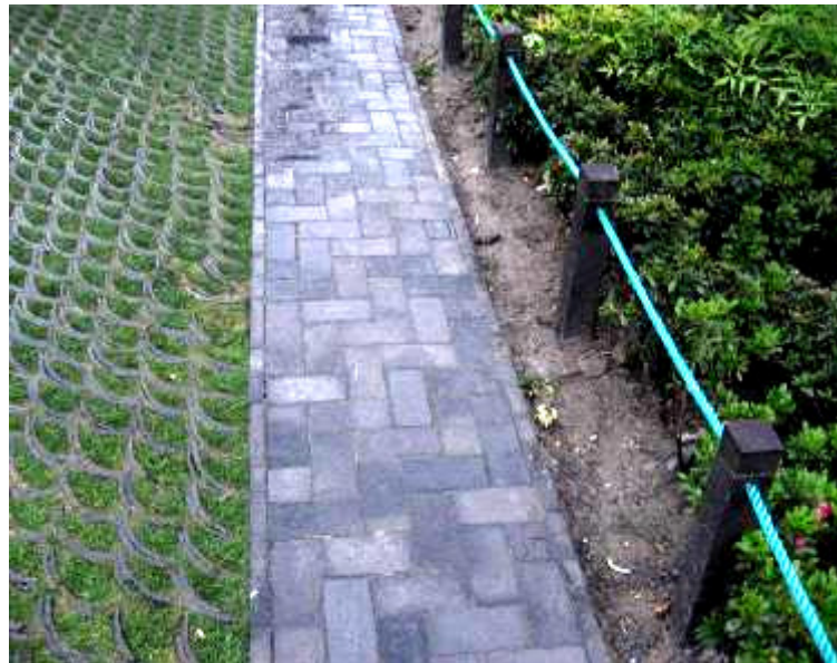
Permeable grass pavers use in sloped seating area with walkway in rough finished stone pavers. (Shanghai)
