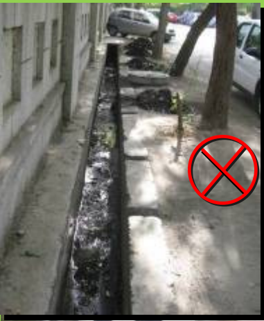
Silted Open Drain, Tughlaqabad Institutional Area
