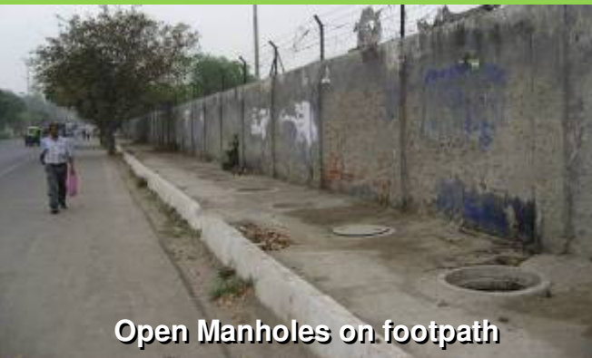
Utilities on Footpath
