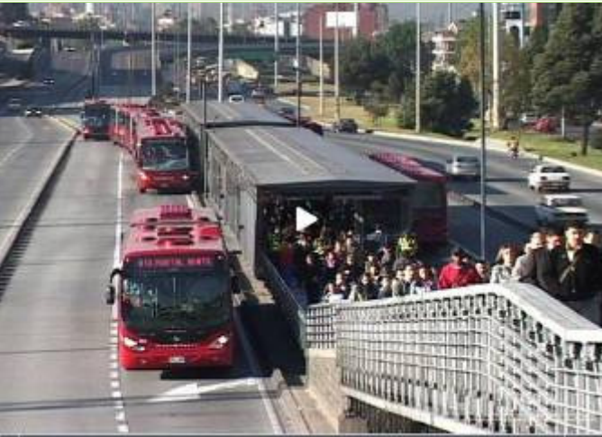
Bogota BRT with segregated median lanes along with express lanes
