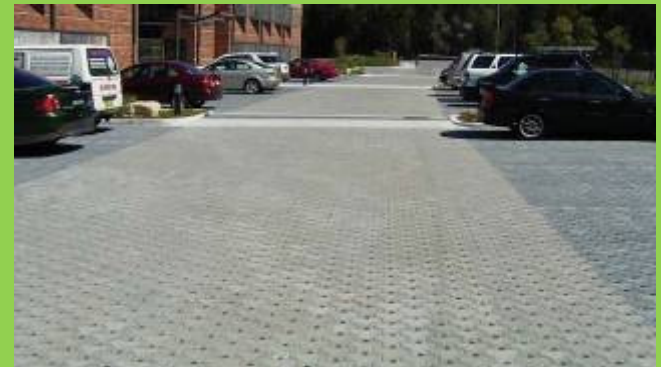
Parking Lot in Sydney, Australia
