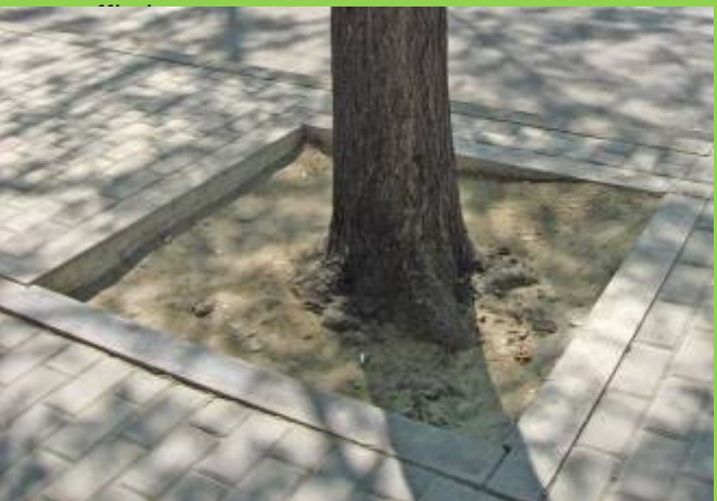
Open Tree pits are acceptable but they are difficult for pedestrians to walk over.
