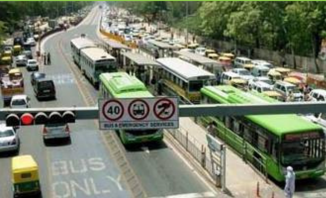
Bus on Segregated BRT Corridor above
