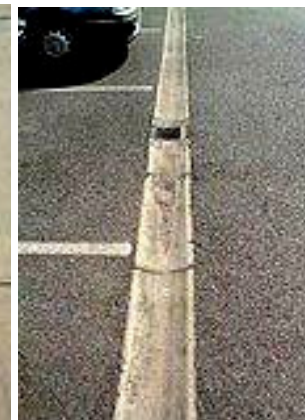
Concrete Drainage Channel in Asphalt Pavement
