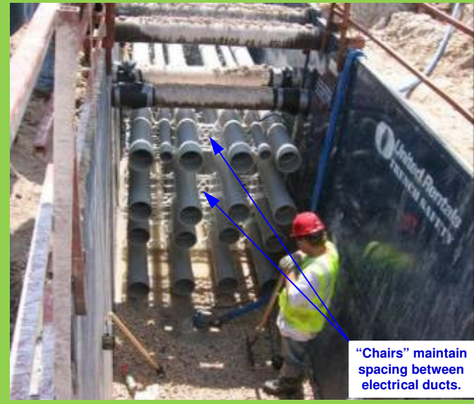
Backfilling the north-south portion of the 5kV electrical duct bank, west of Dupuis Hall
