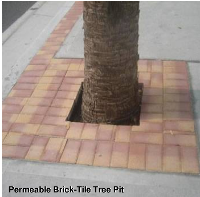
Permeable Cement-Tile Tree Pit
