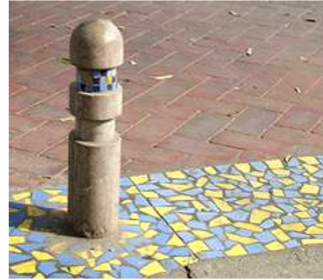
Red tinted PCC Tiles and concrete bollards with glaze Ceramic tile highlights. (BRT Delhi)
