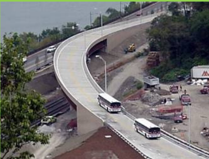
Dedicated Bus ramp
