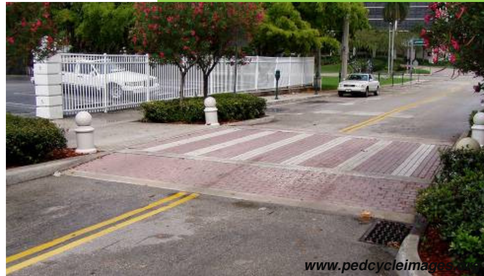
Only Anti-Skid, uniform materials to be used on Tabletop Crossings – for comfortable access by people with reduced mobility.
