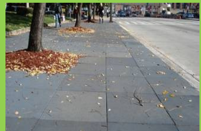
Permeable Rubber Sidewalk in Vancouver
