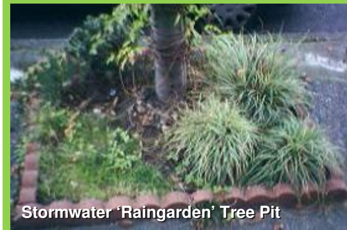
Permeable Cement-Tile Tree Pit
