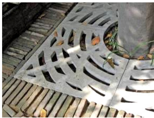
Sample Detail of Precast Cement Concrete Tree Grating.
