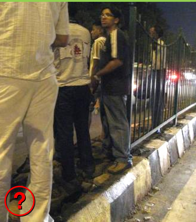
Inadequate, unusable refuge island at a signalized intersection in ITO
