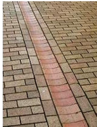
Brick Drainage Channel in Walkway
