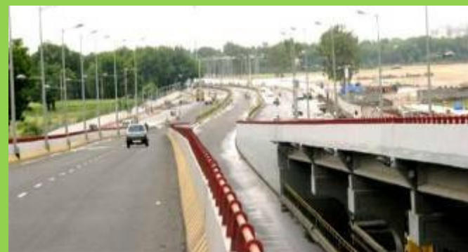
Treatment of existing flyover at Ahmedabad.
