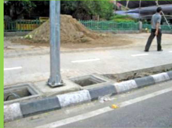
Utilities along the 0.7 M Buffer Zone between Cycle Path and MV Lane, BRT corridor, Delhi.
