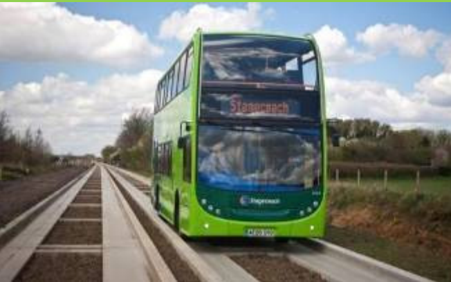
Kerb guided busway at Cambridge UK
