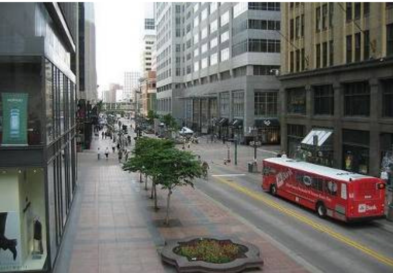
Nicolett Street transit mall, Minneapolis with extra wide sidewalks created by removing through lanes.
