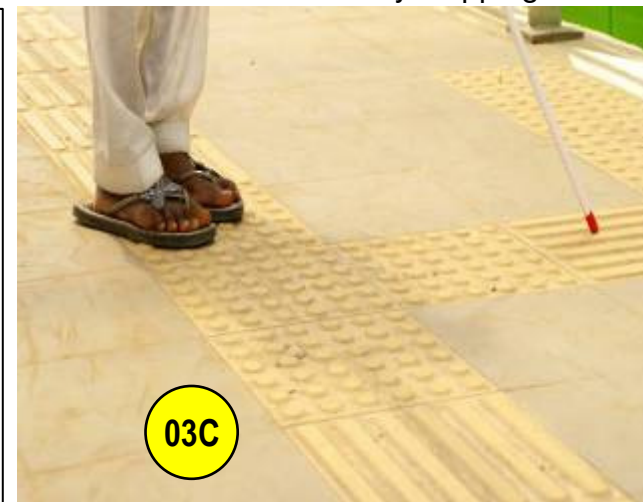
Engineering configuration of floor tactile tiles
