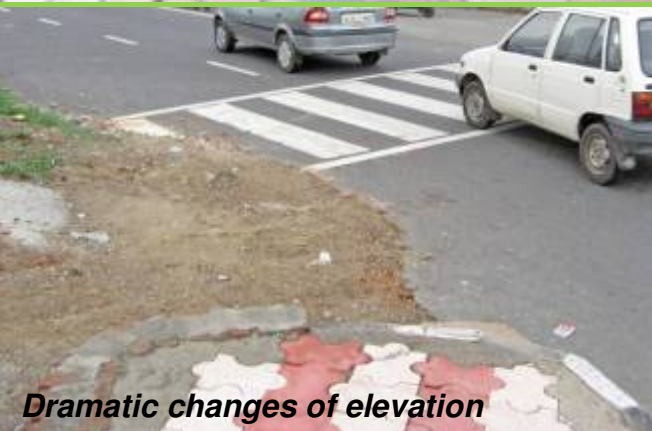
Uneven pavement surface due to lack of proper setting in a concrete sub-base.
