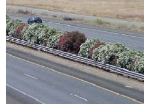
Three beams as barrier
