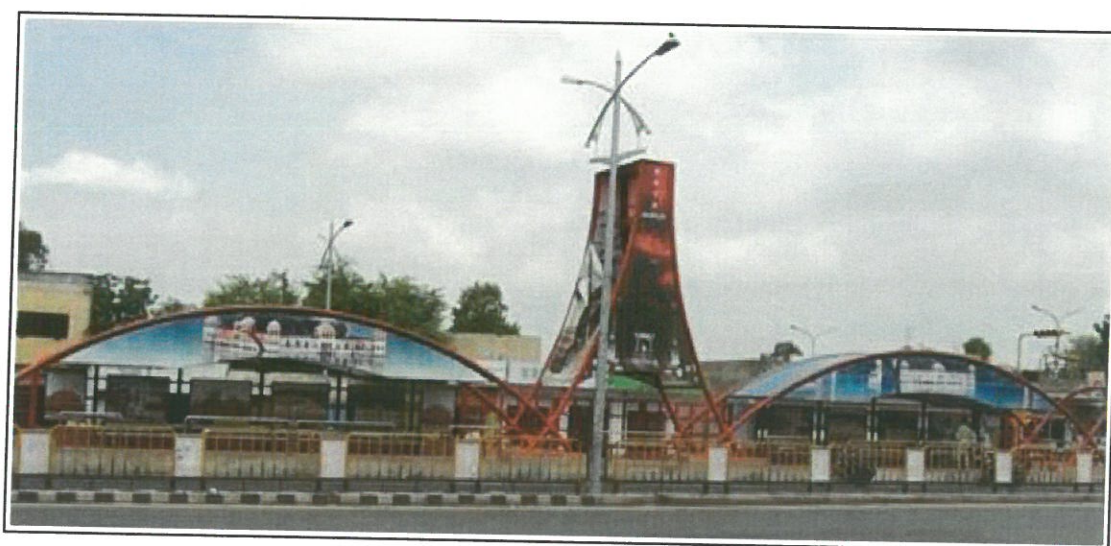
Figure 3.3: View of Bus Station / Stop on BRTS Corridor
