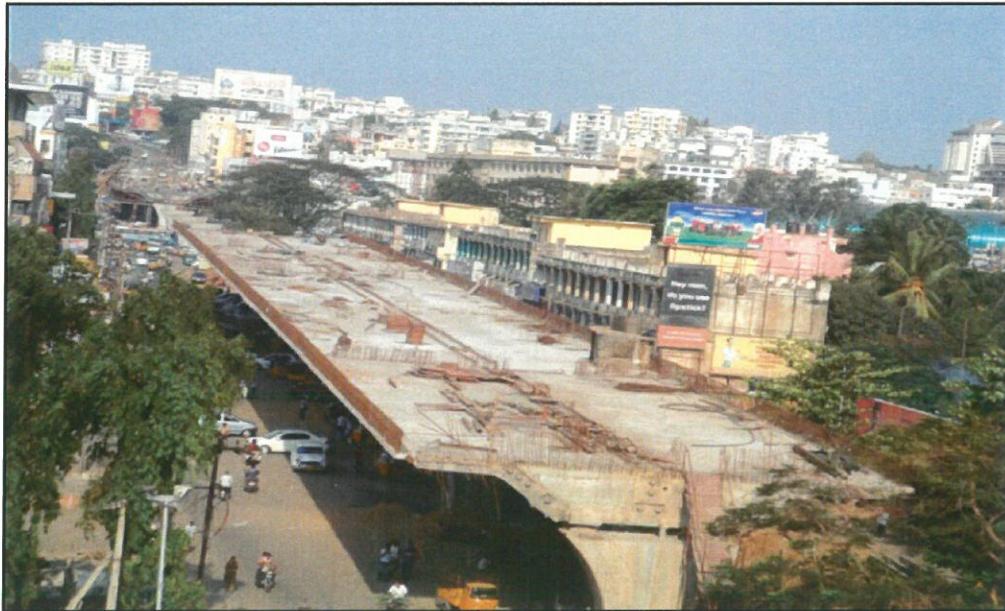
Figure 11.9: Flyover in Progress at Visakhapatnam
