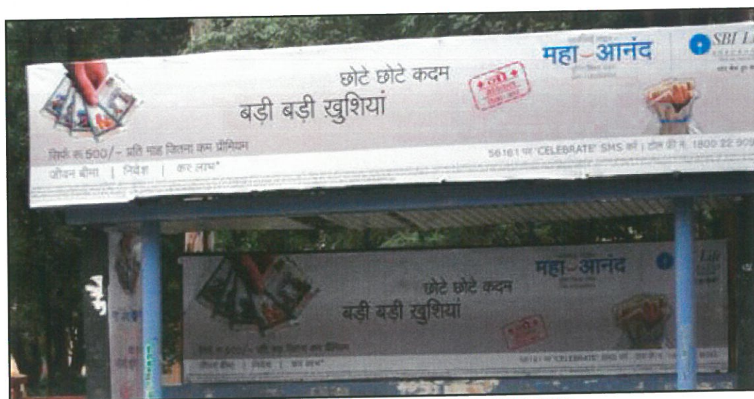
Figure 5.2: Metro Bus Service Shelter, JCTSL 2010
