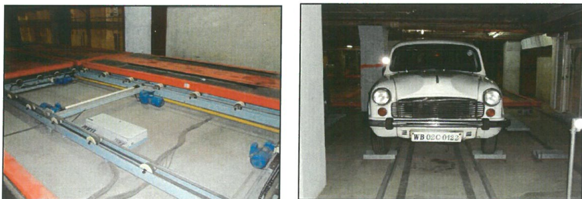
Figure 10.3: Types of Parking: a) Palette Shifting and b) Shuttle
