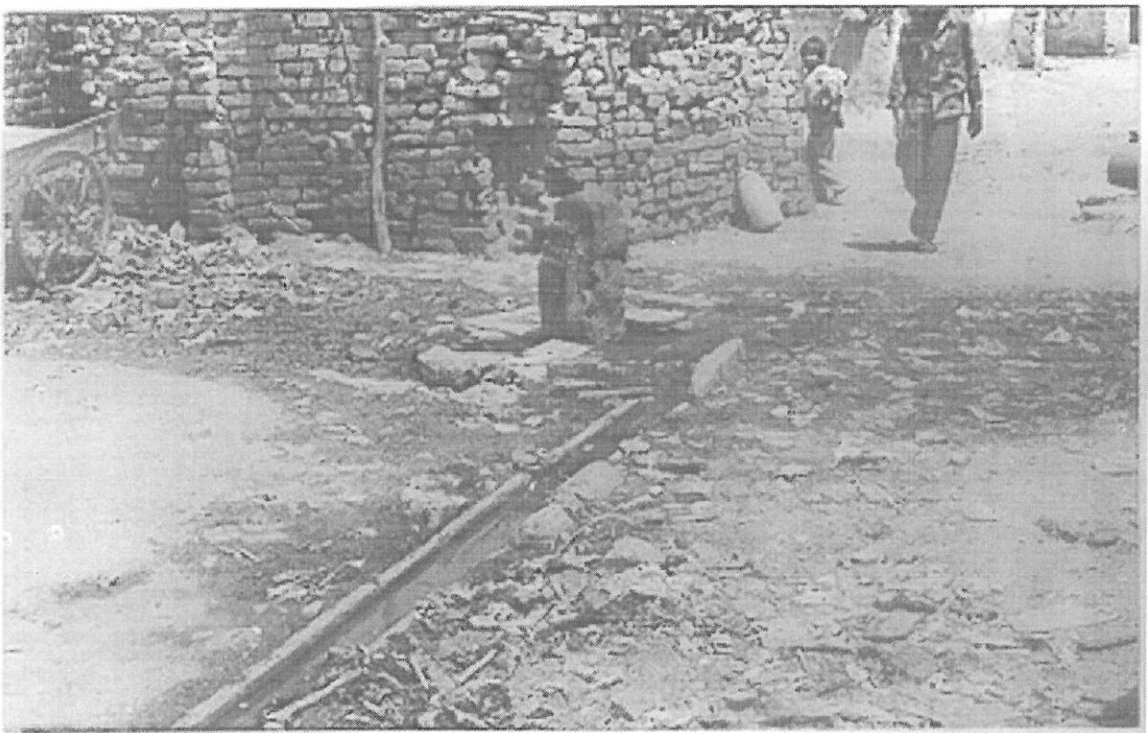
Condition of open drains in the urban slums
