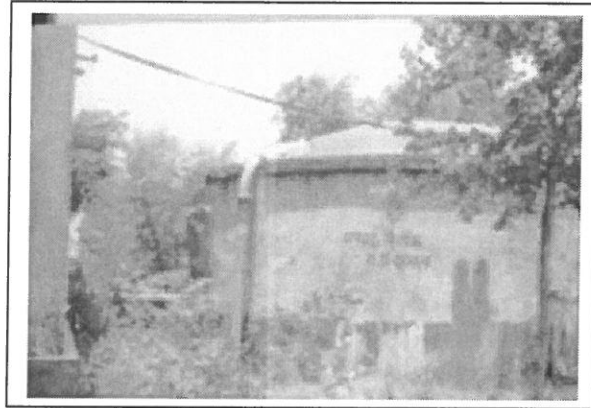
Photograph 36: View of CWR constructed prior to implementation of AUWSP
