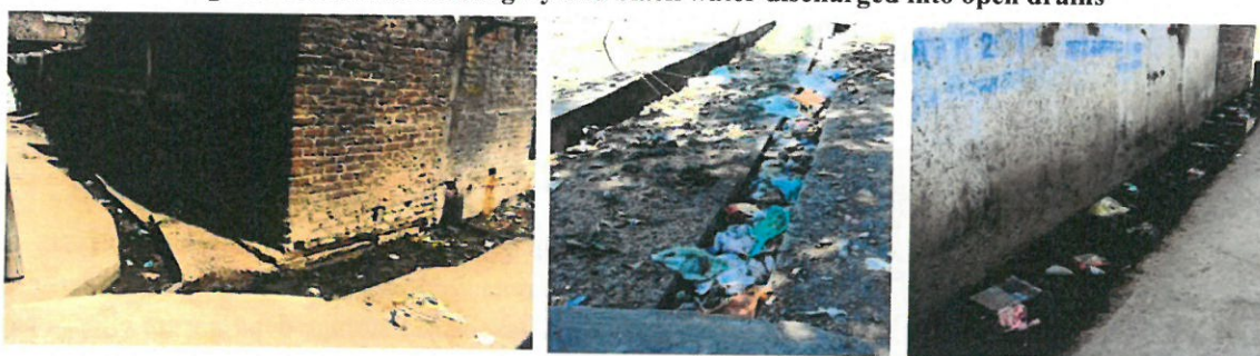
Figure 2: Household level grey and black water discharged into open drains
