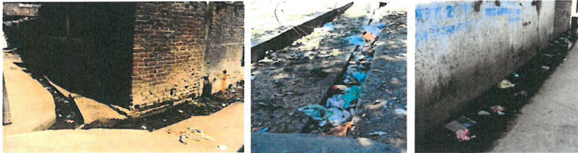
Figure 3: Household level grey and black water discharged into open drains
