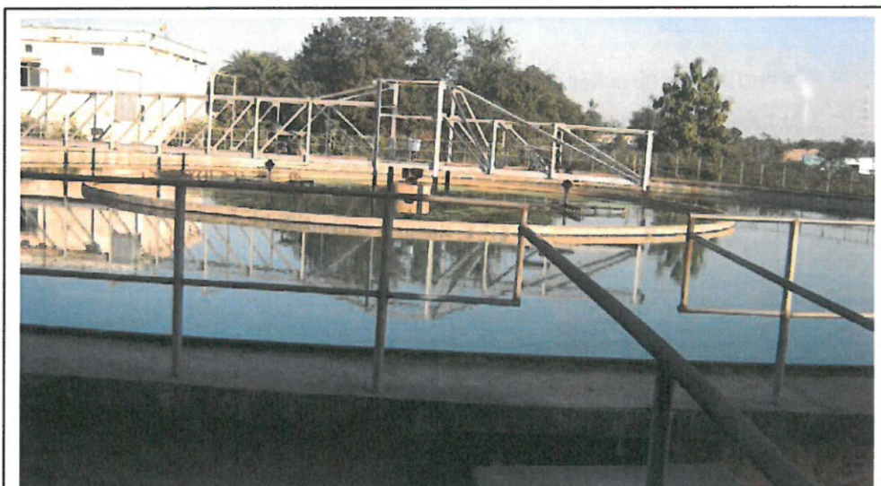
55 MLD WTP at Rourkela
