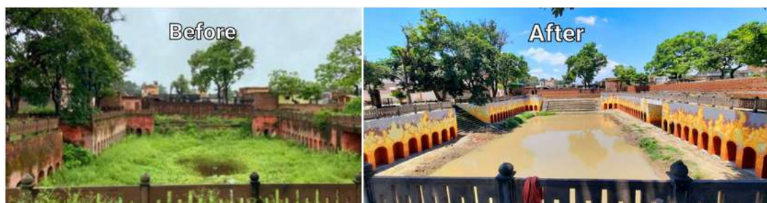
Image 12: Status of a kund in Ayodhya before and after rejuvenation
